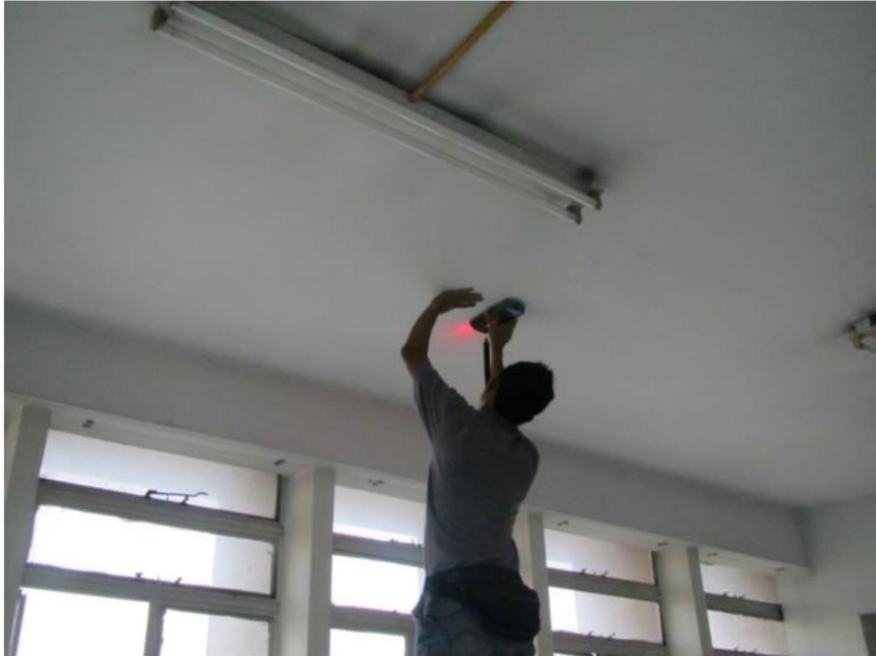
Scanning the rebar
