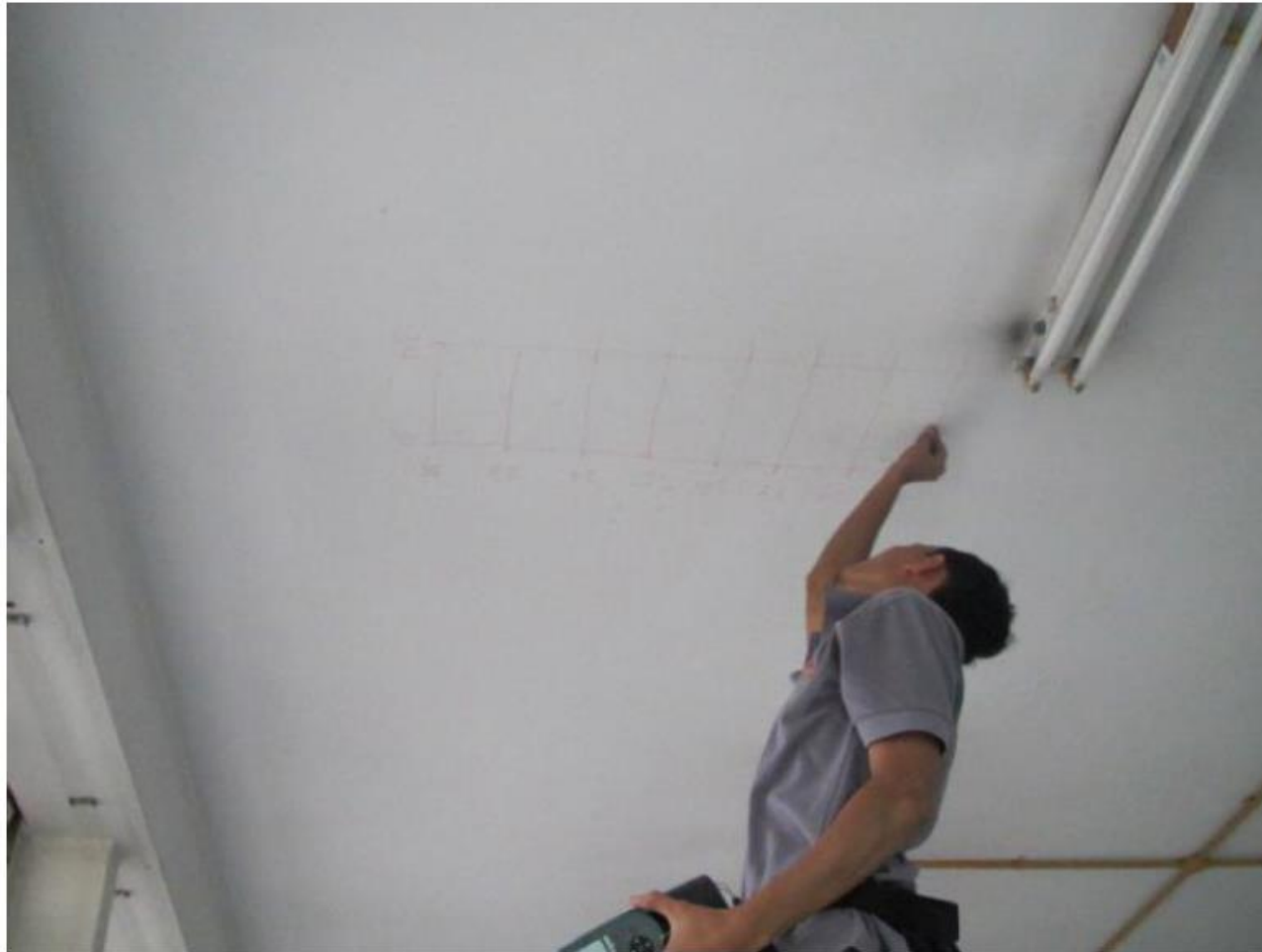
Marking the testing grid
