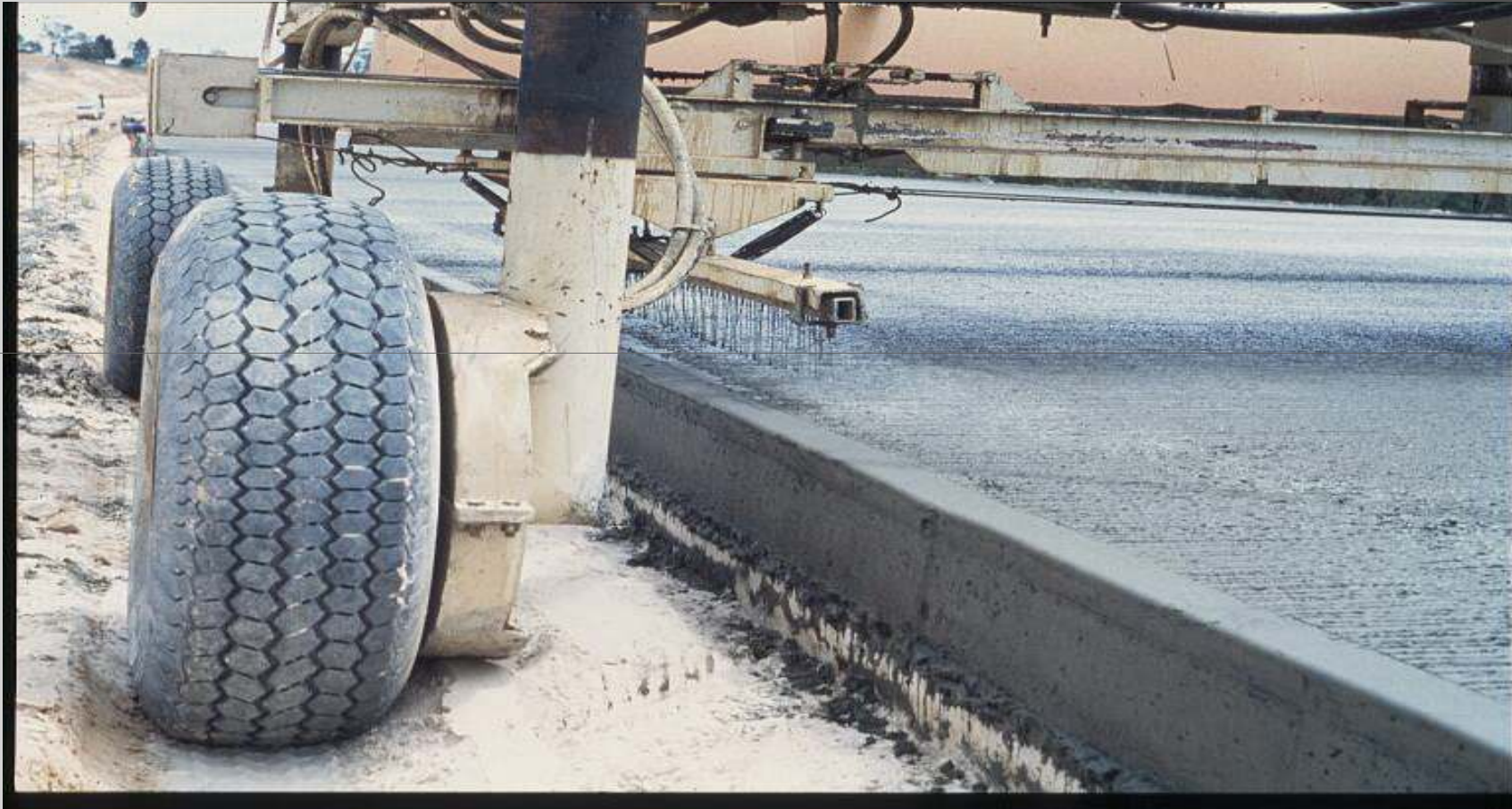
Texturing device, showing spring steel tynes on “broom”
