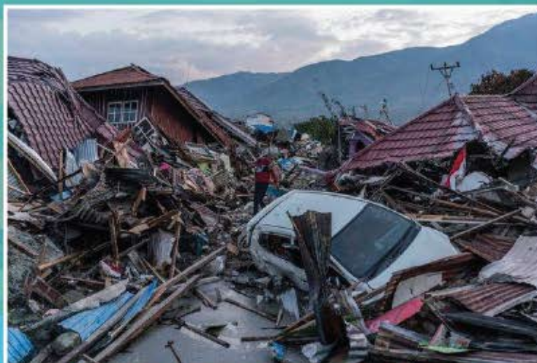
A destroyed neighbourhood in Palu, Indonesia due to liquefaction
