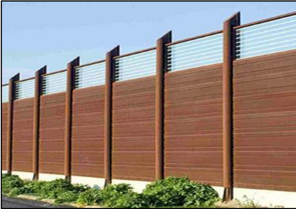
Figure 1.8: Wood Noise Barrier
