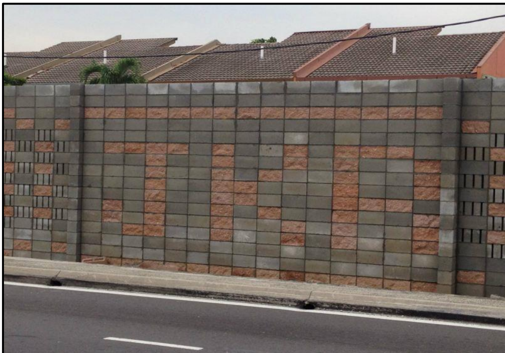
Figure 1.5: Masonry Noise Barrier
