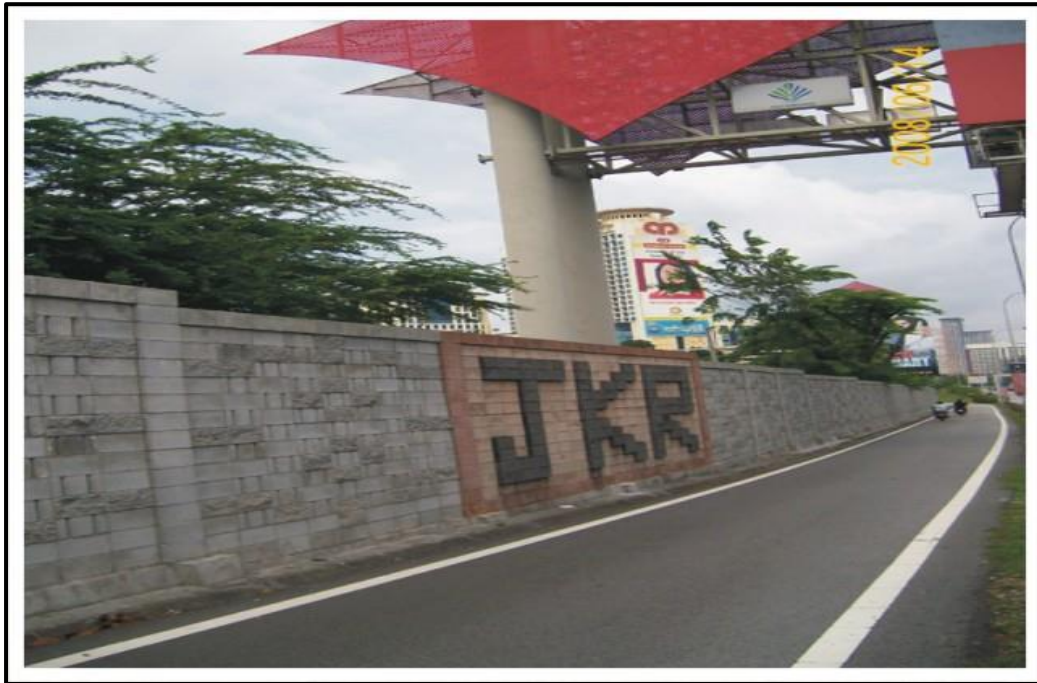
Figure 1.4: Masonry Noise Barrier at Federal Highway
