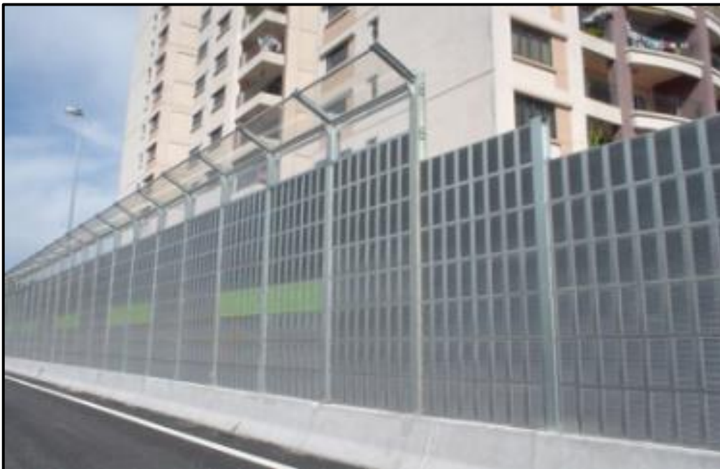
Figure 1.7: Metal Noise Barrier
