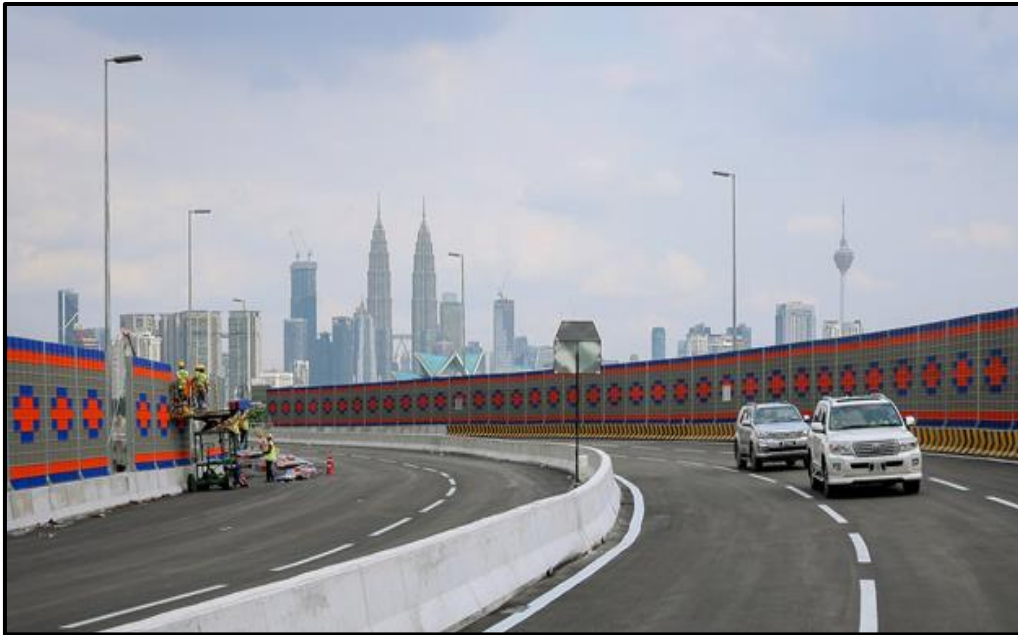
Figure 1.6: Metal Noise Barrier at Duta-Ulu Kelang Expressway Phase 2 (DUKE)
