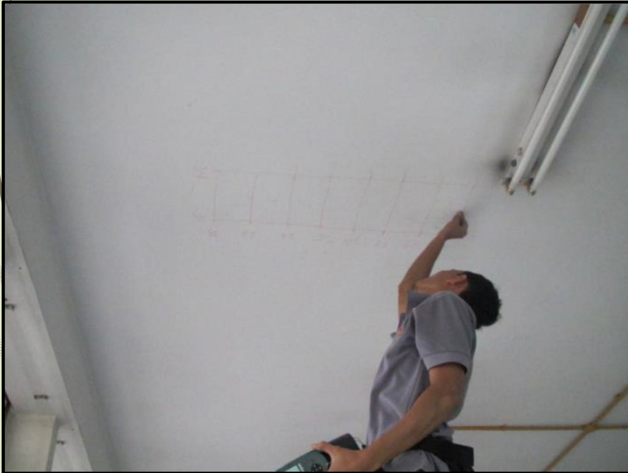
Marking the testing grid
