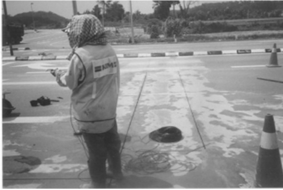
Install Traffic Signal Loop Detector
