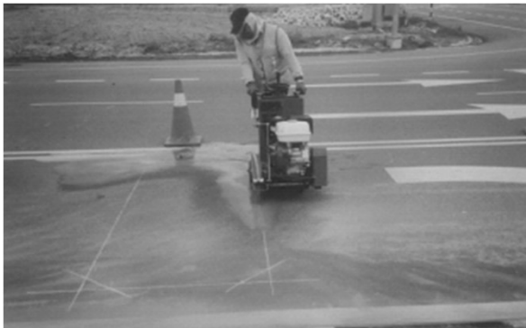
Install Traffic Signal Loop Detector
