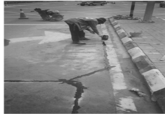
Install Traffic Signal Loop Detector
