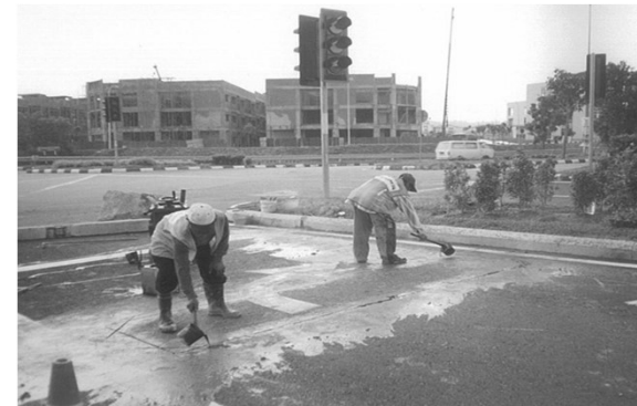
Install Traffic Signal Loop Detector
