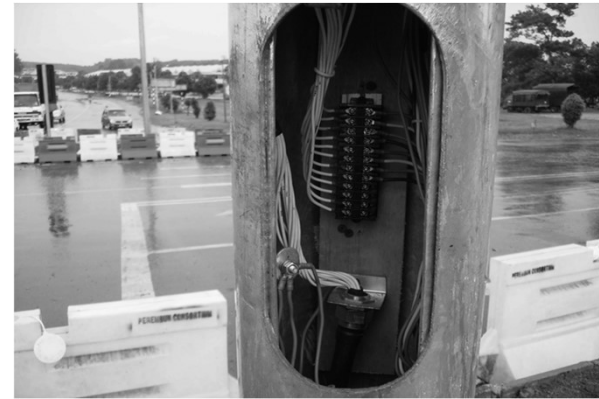
• Termination Signal Cable On Traffic Pole
