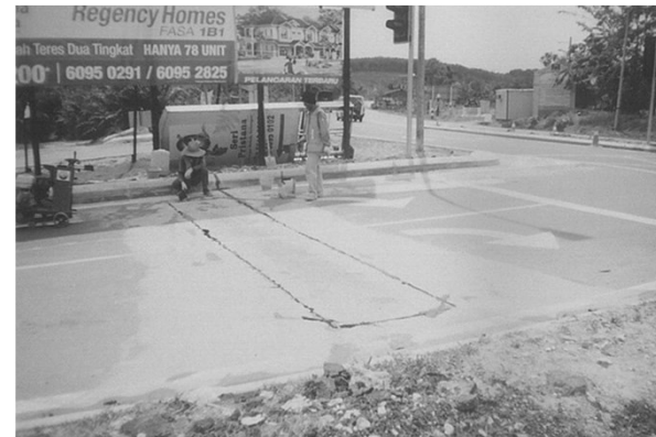
Install Traffic Signal Loop Detector
