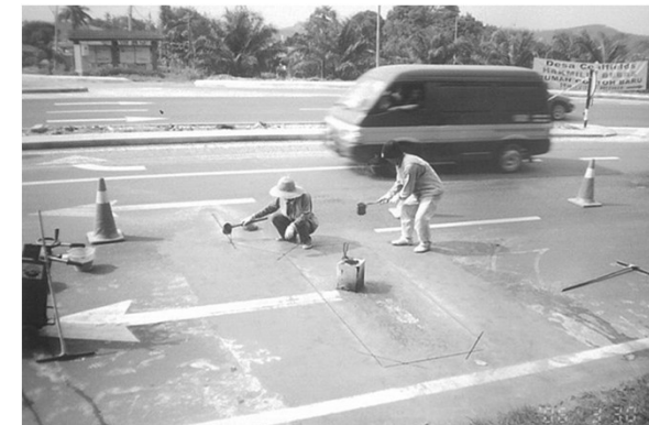
Install Traffic Signal Loop Detector
