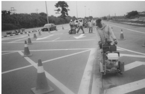
Install Traffic Signal Loop Detector
