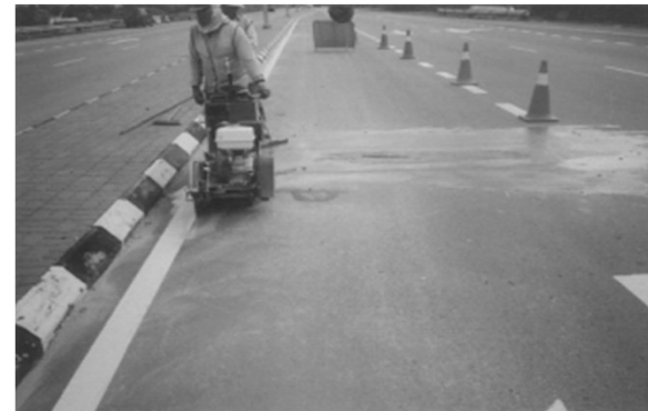
Install Traffic Signal Loop Detector
