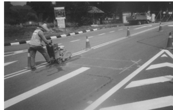
Install Traffic Signal Loop Detector
