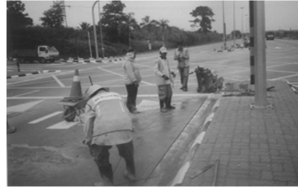
Install Traffic Signal Loop Detector
