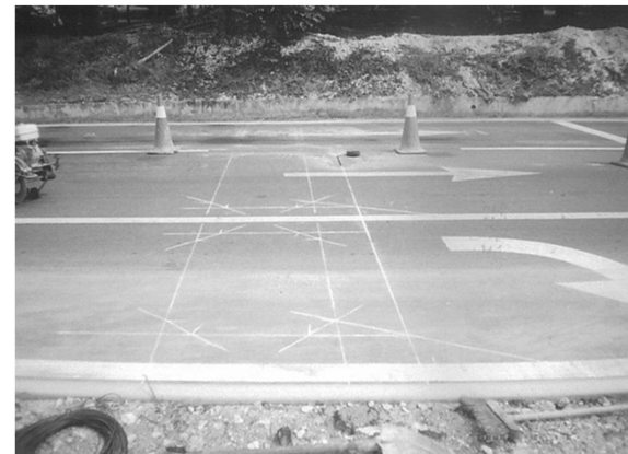
Install Traffic Signal Loop Detector
