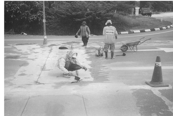
Install Traffic Signal Loop Detector
