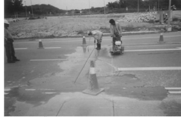
Install Traffic Signal Loop Detector
