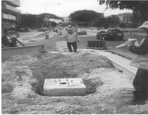
Traffic Signal Overhead Pole (Mast Arm) Plinth
