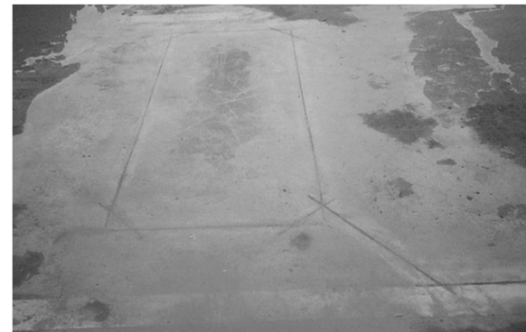
Install Traffic Signal Loop Detector
