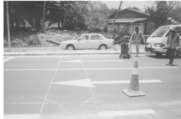
Install Traffic Signal Loop Detector
