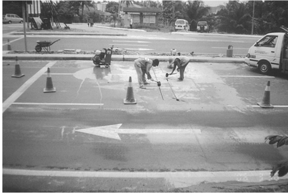
Install Traffic Signal Loop Detector
