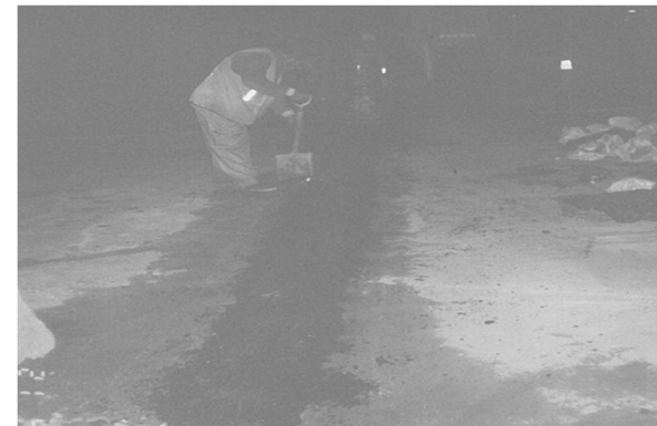
• Laying G.I Pipe on Carriageway
