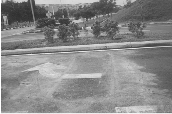
Install Traffic Signal Loop Detector
