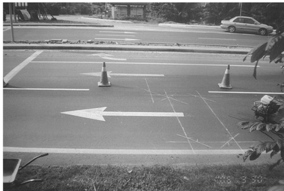
Install Traffic Signal Loop Detector
