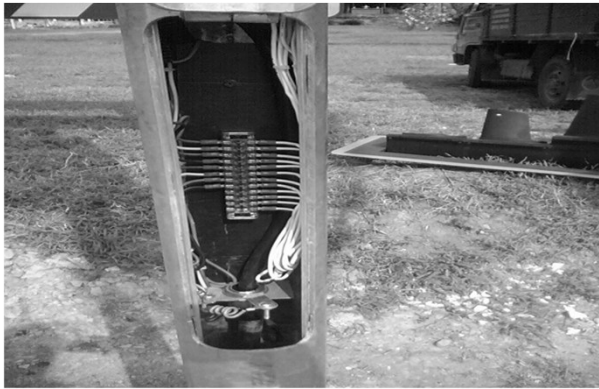
Termination Signal Cable On Traffic Pole
