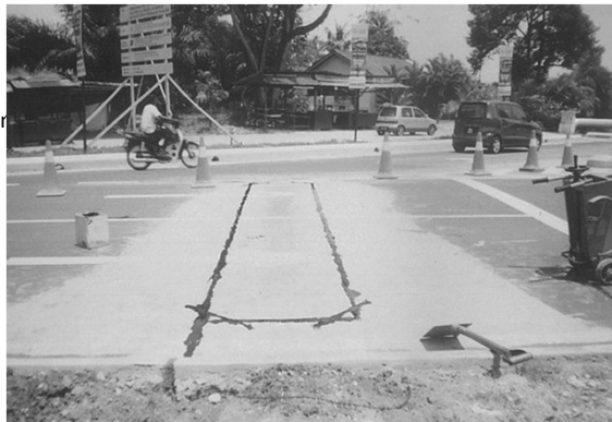
Install Traffic Signal Loop Detector
