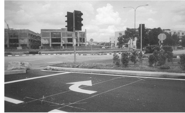
Install Traffic Signal Loop Detector
