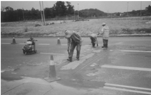
Install Traffic Signal Loop Detector
