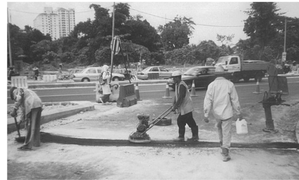
• Laying G.I Pipe on Carriageway
