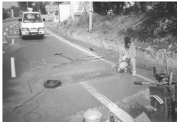
Install Traffic Signal Loop Detector
