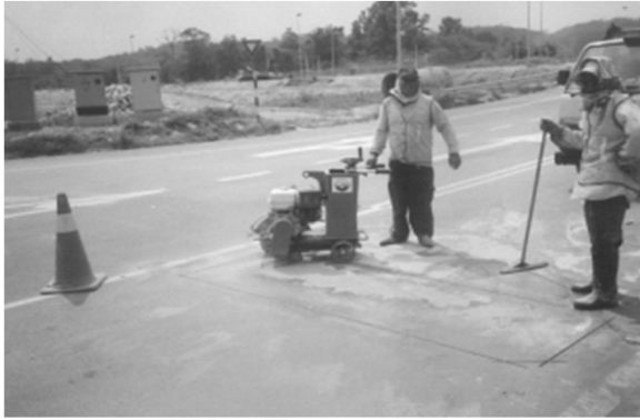
Install Traffic Signal Loop Detector
