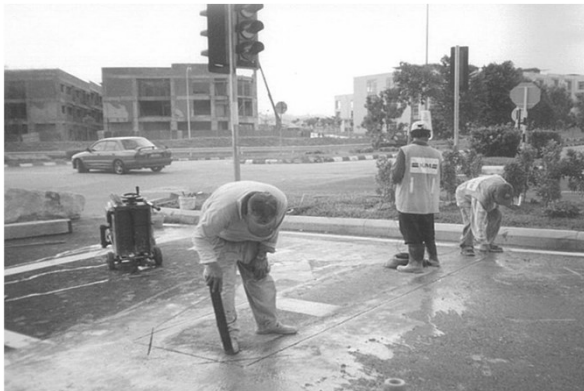
Install Traffic Signal Loop Detector
