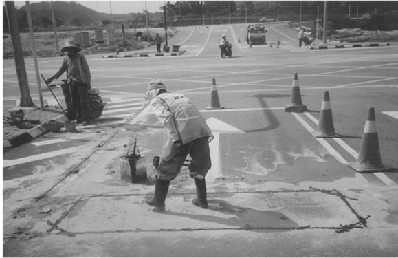
Install Traffic Signal Loop Detector
