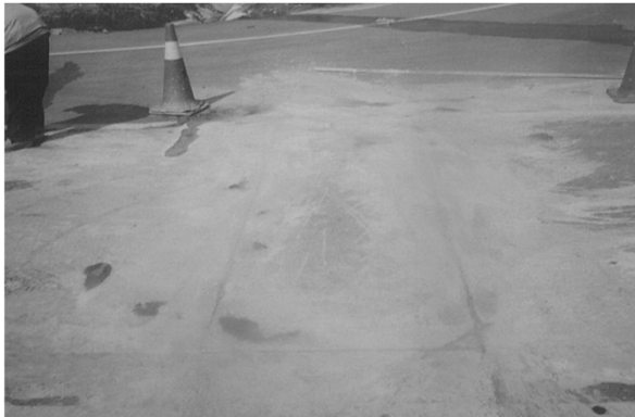
Install Traffic Signal Loop Detector
