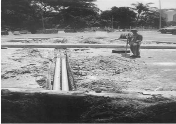
Laying G.I Pipe on Carriageway
