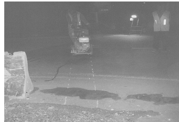
Saw cut on carriageway
