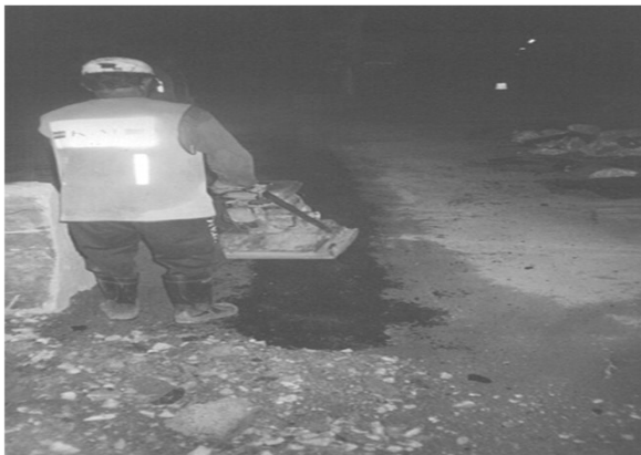
• Laying G.I Pipe on Carriageway
