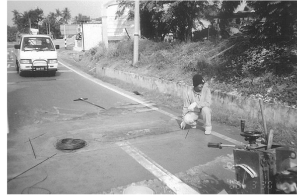
Install Traffic Signal Loop Detector
