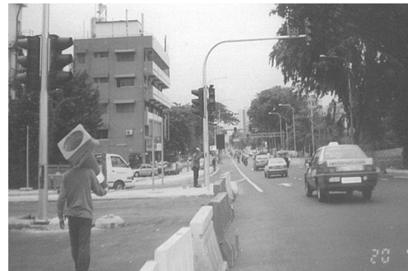
• Traffic Signal Overhead Pole (Mast Arm)
