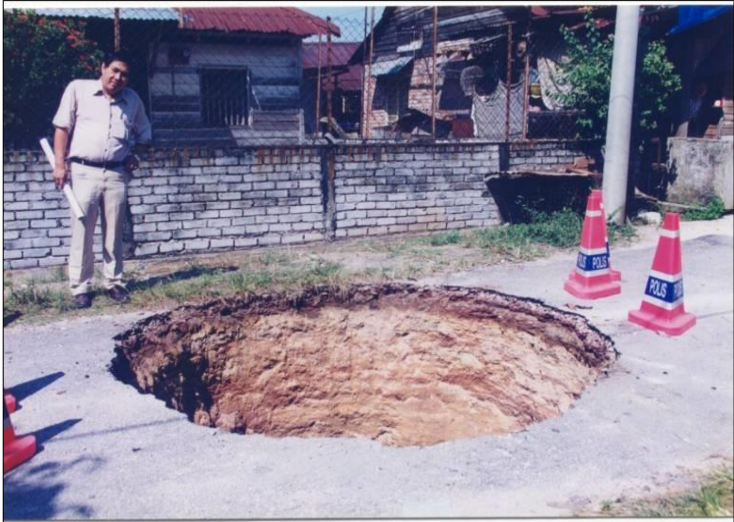
Sinkhole occurrence in limestone area
