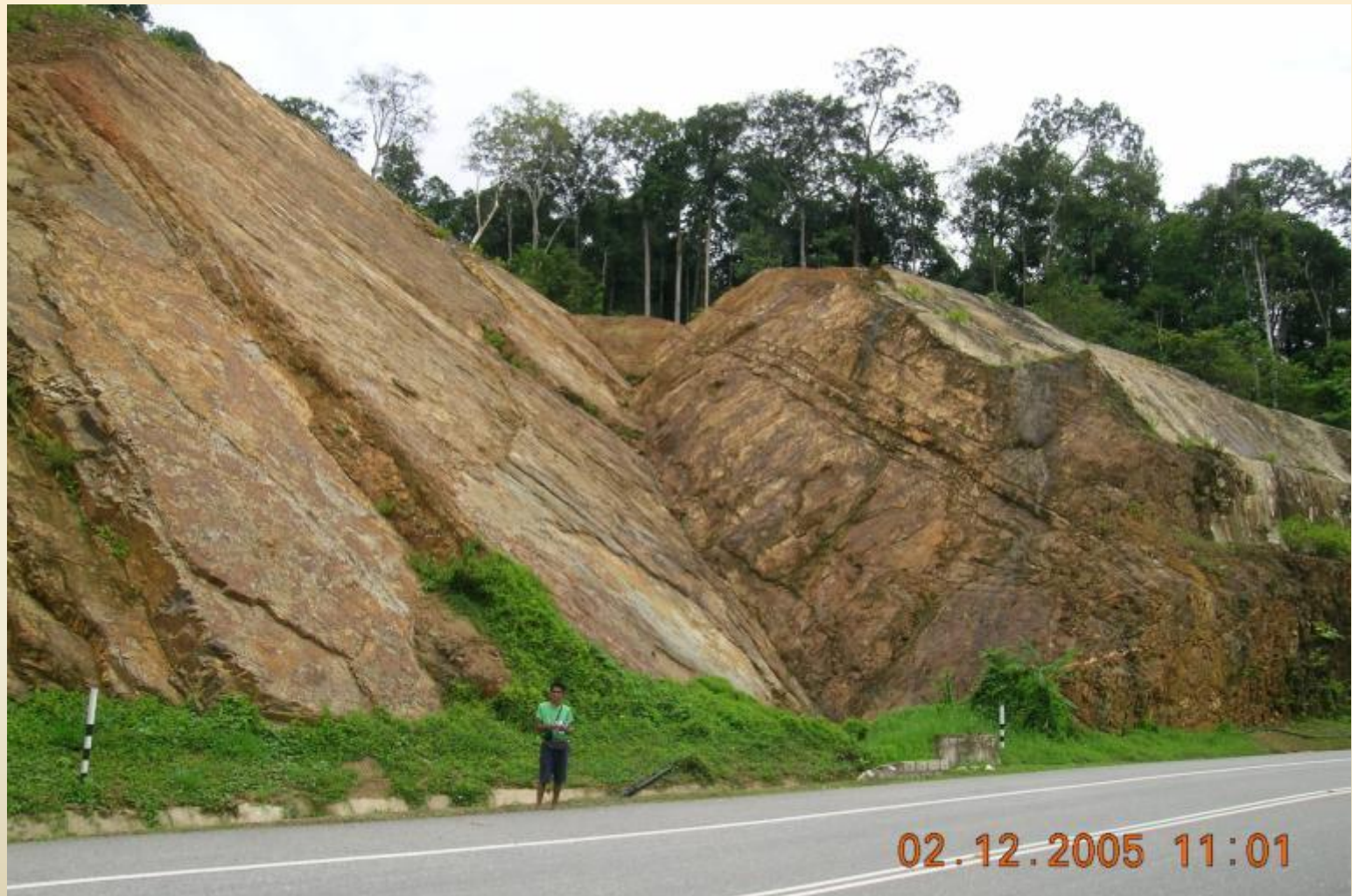
A typical example of wedge failure at Cameron Highland Gua Musang Road
