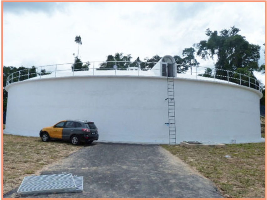
Tangki Simpanan Air Berkapasiti 1,500,000 Gallon
