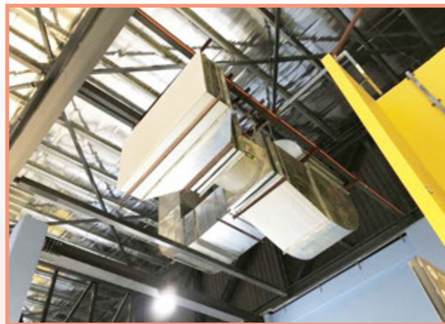
Sistem Smoke Spill Extractor
