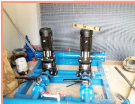
Elevated Water Storage Tank Di Tapak
