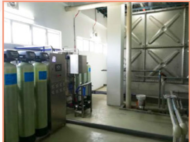
Sistem Reverse Osmosis Water Dan Storage Water Tank Di Aras Tangki
