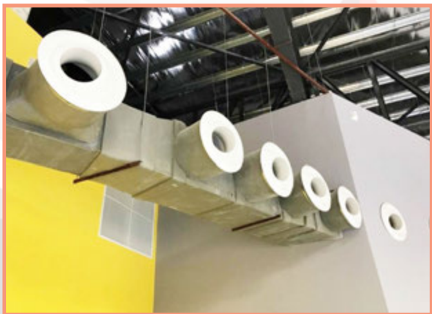
Jet Diffuser Dipasang Mengikut Arah Putaran Trek Basikal
