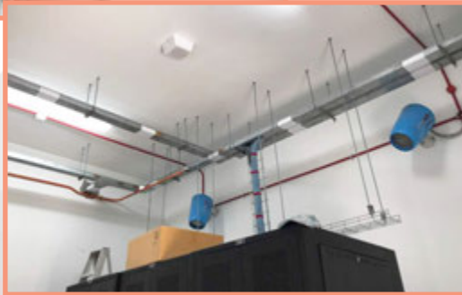
Sistem Pencegah Kebakaran (Clean Agent System)
