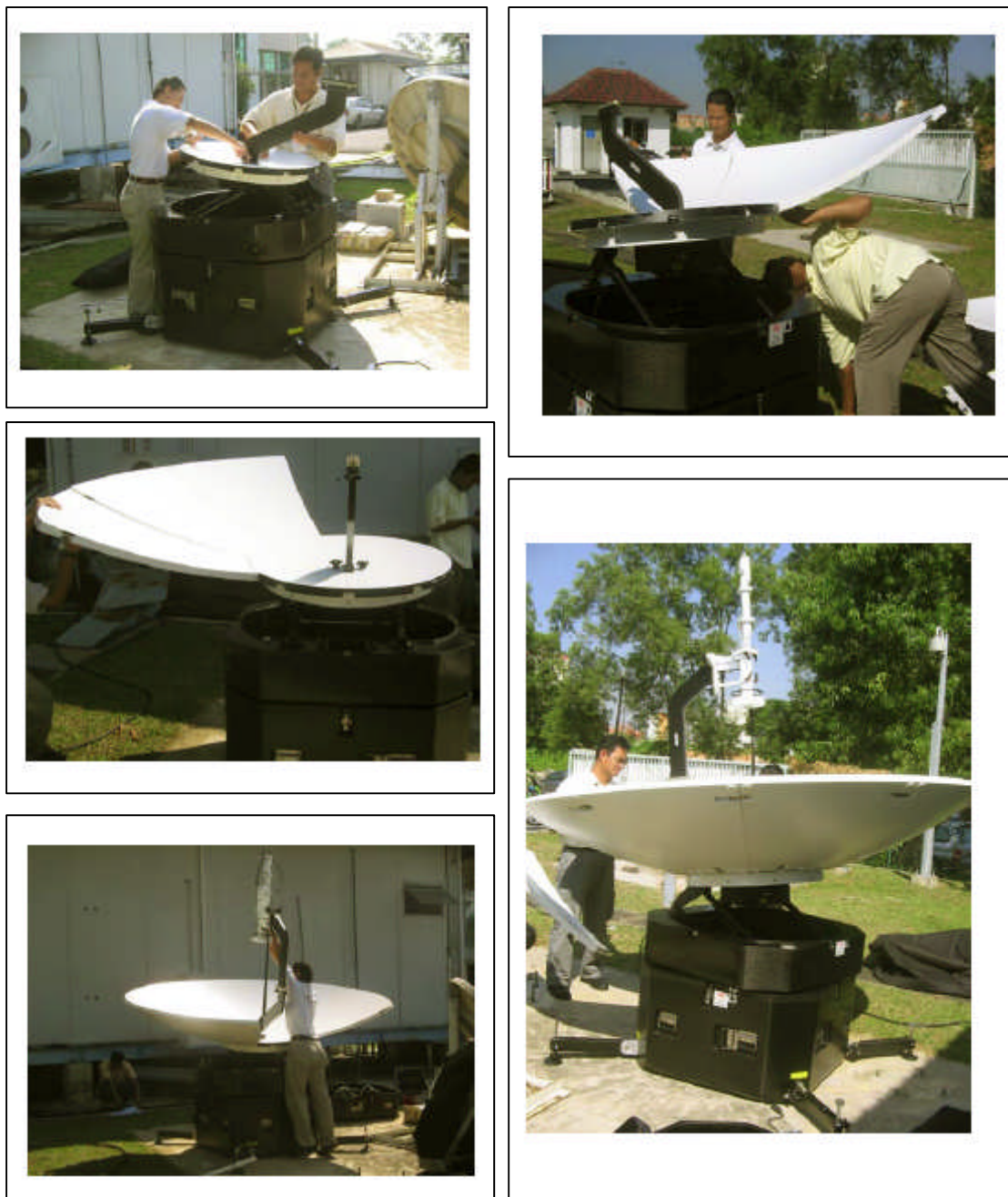
Figure 9.26: Installation of flyaway antenna
