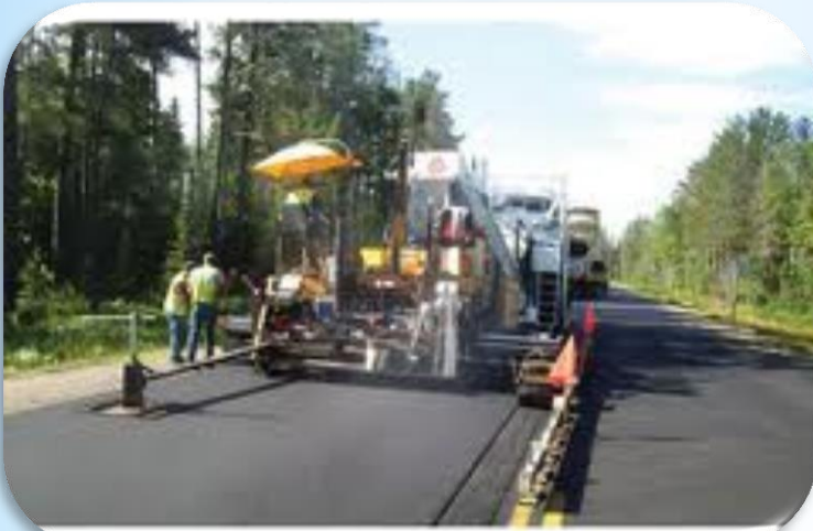
Resurfacing (Mill and Pave)
