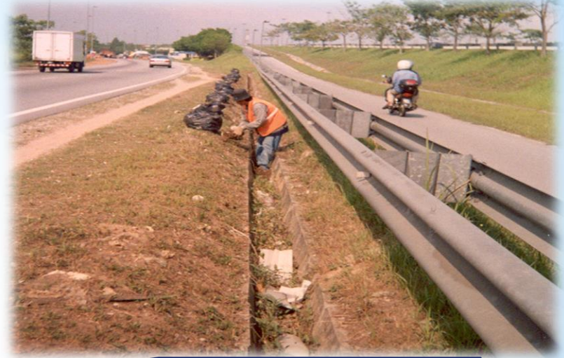
Cleaning of drains
