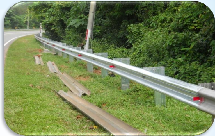
Guardrail Replacement
