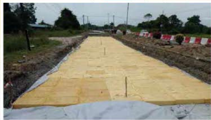
Figure 3. The concept of polyurethane flatbed application for construction of new roads.
