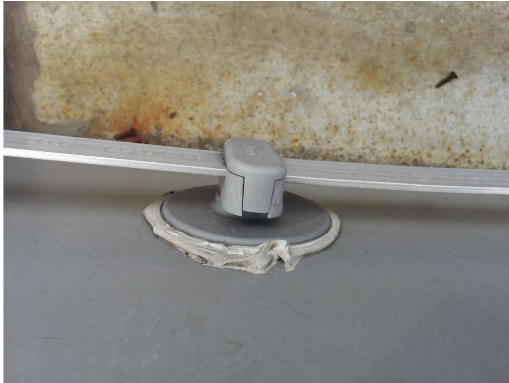
Adhesive DC tape clip Use on metal deck roof
