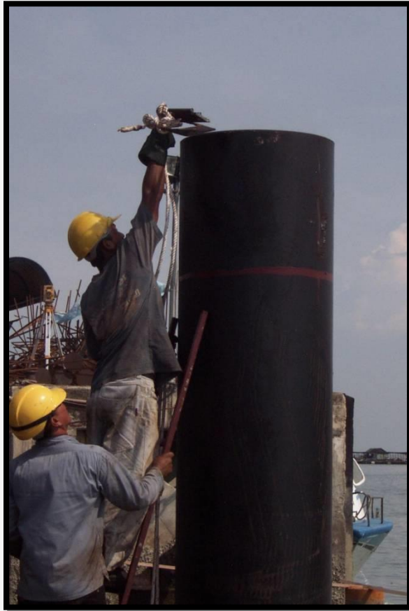
Proses penanaman Tide Well semasa pembinaan STAPS Kukup (2005)
