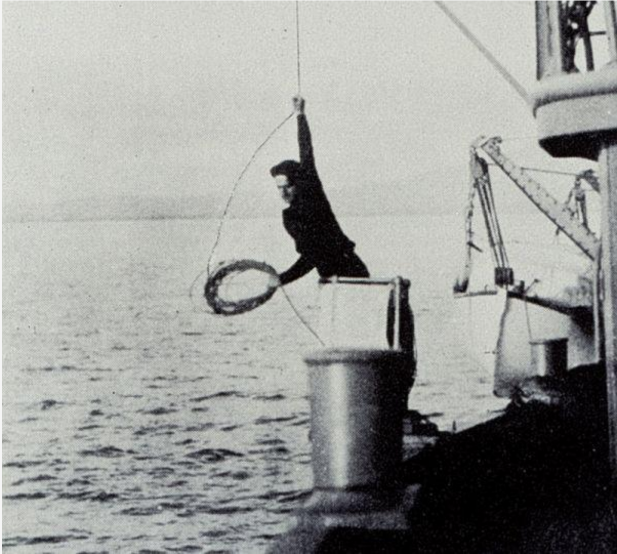
Leadline sounding operation. (Photo: 1928 and 1931, Hydrographic Manual)
