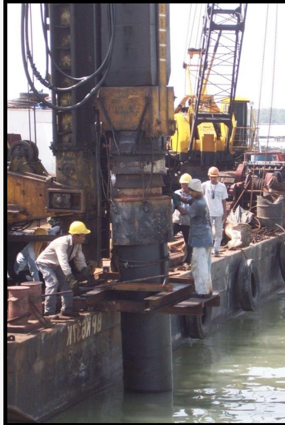
Proses penanaman Tide Well semasa pembinaan STAPS Kukup (2005)
