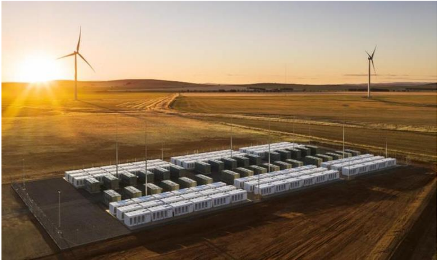
The 100 MW lithium-ion energy storage system by TESLA. The largest ESS in the world
