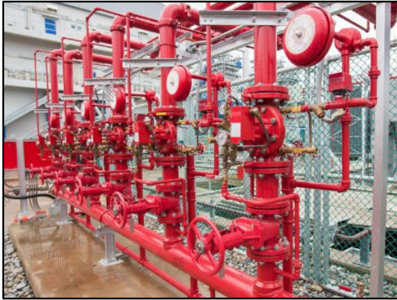
GAMBAR 1.3: CONTOH PEMASANGAN INSTALLATION CONTROL VALVE
