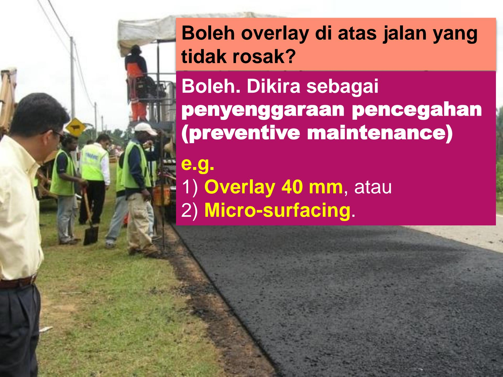
A photograph showing a construction site where workers in yellow vests are applying asphalt overlay to a road. One worker is standing on a lift, spreading asphalt, while others stand by. A yellow 'Caution' sign is visible in the background. The new asphalt surface is dark grey and appears smooth.
