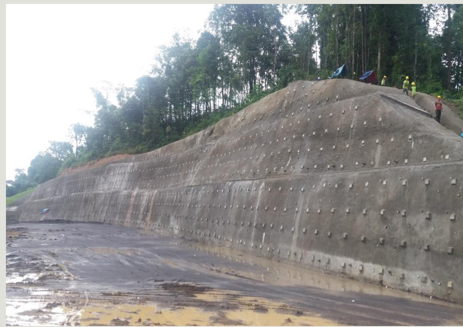
KERJA GUNITING DAN SOIL NAILING
