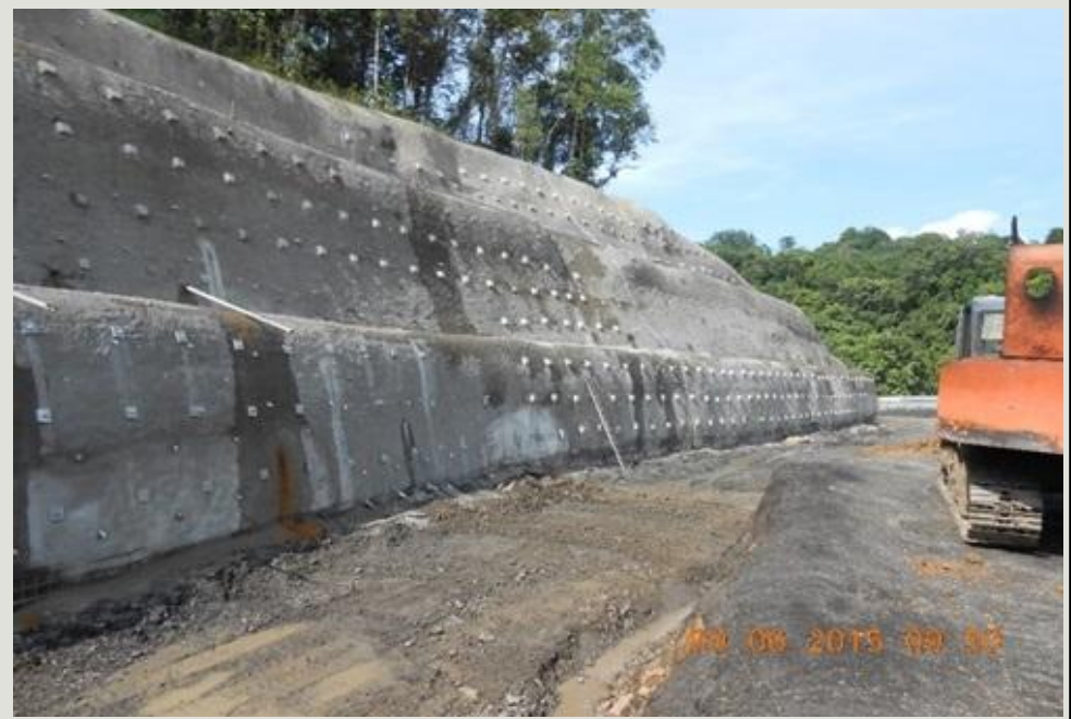
KERJA GUNITING DAN SOIL NAILING
