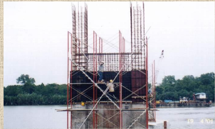
Installation of steel form
