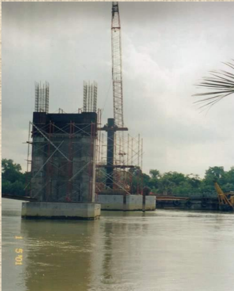
Staging & formwork preparation
