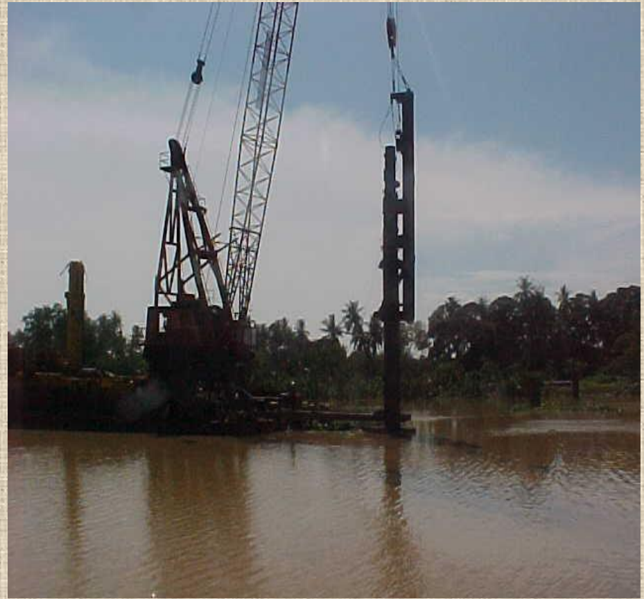
Pile driving-hydraulic hammer
