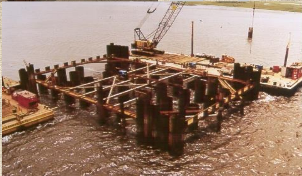
Membina Coffer Dam Di kawasan Perairan
