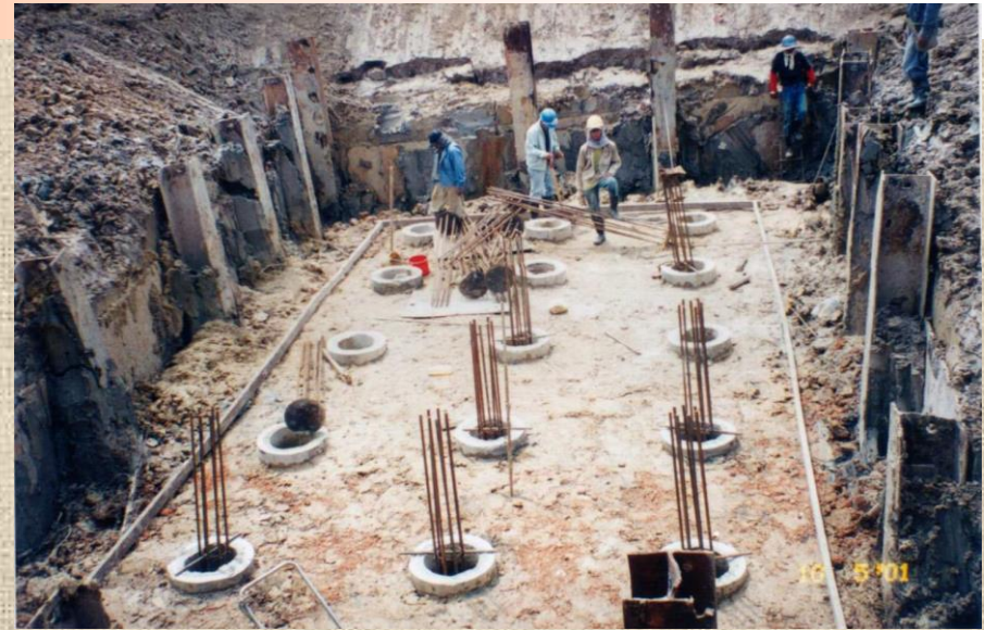
Pile plug rebar
