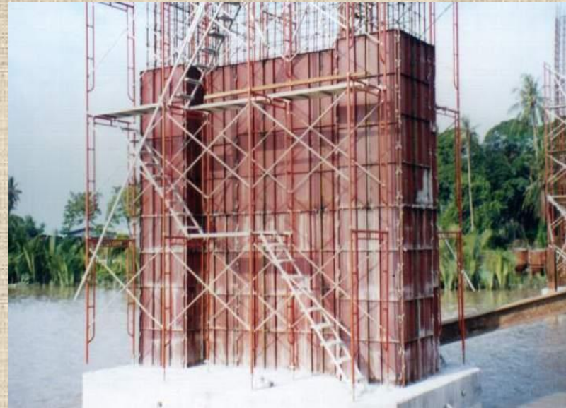
Casting of piers in stages
