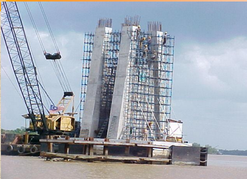
Staging & casting of pylon's pier Installed fender system at pile cap sides
