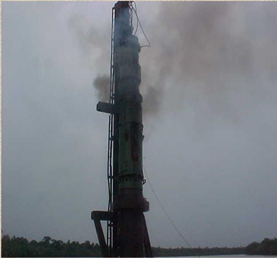
Pile driving-hydraulic hammer
