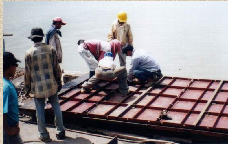
Casting of piers in stages
