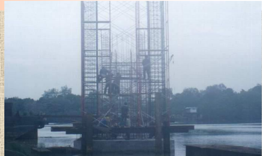
Rebar for pier P2
