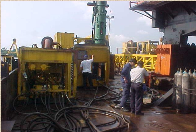
Equipments on barge
