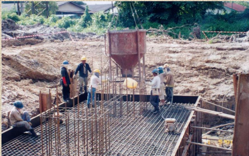
Concreting pile cap
