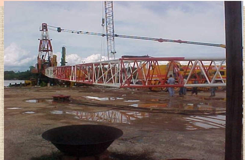
Barge for piling rig
