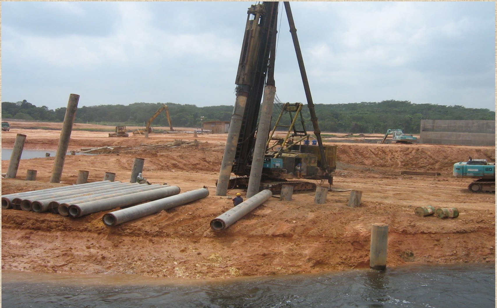
Kerja Penanaman Raked Spun Piles
