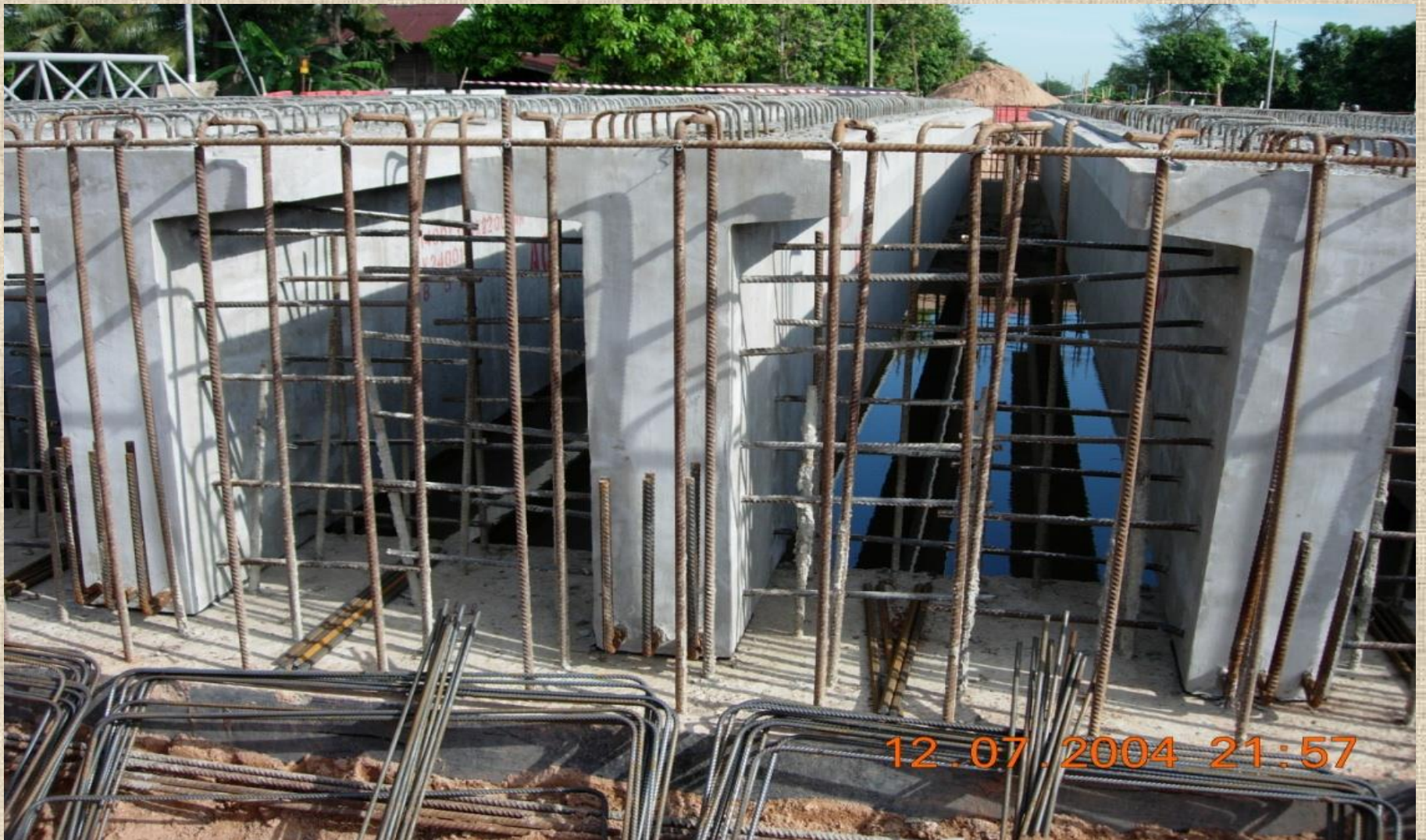
Rebars ;Continuity End Diaphragm
