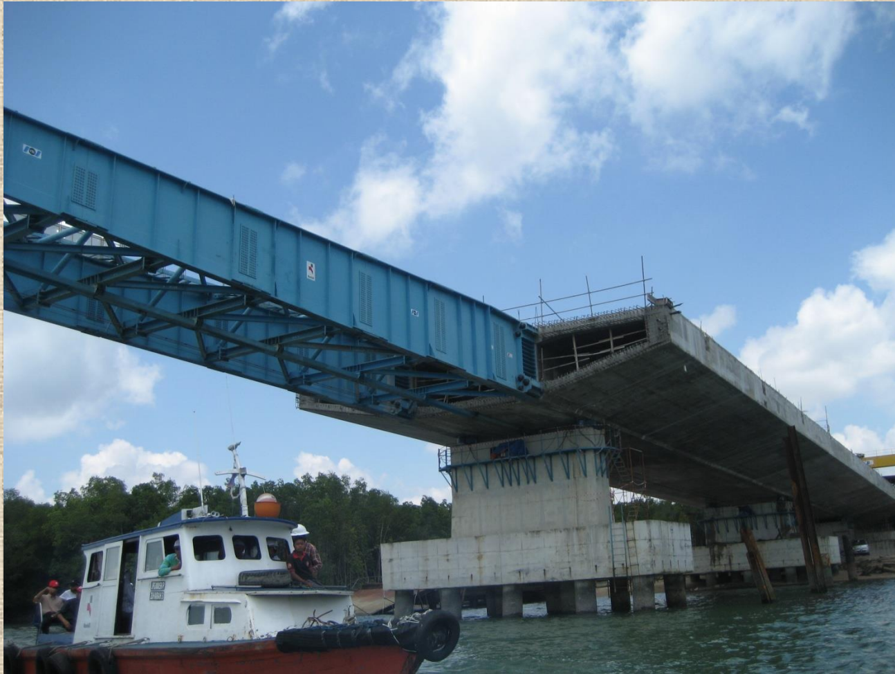
Pile Cap Above High Tide Level
