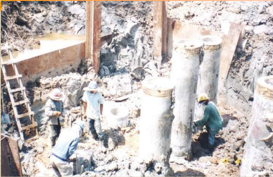
Cutting of pile head
