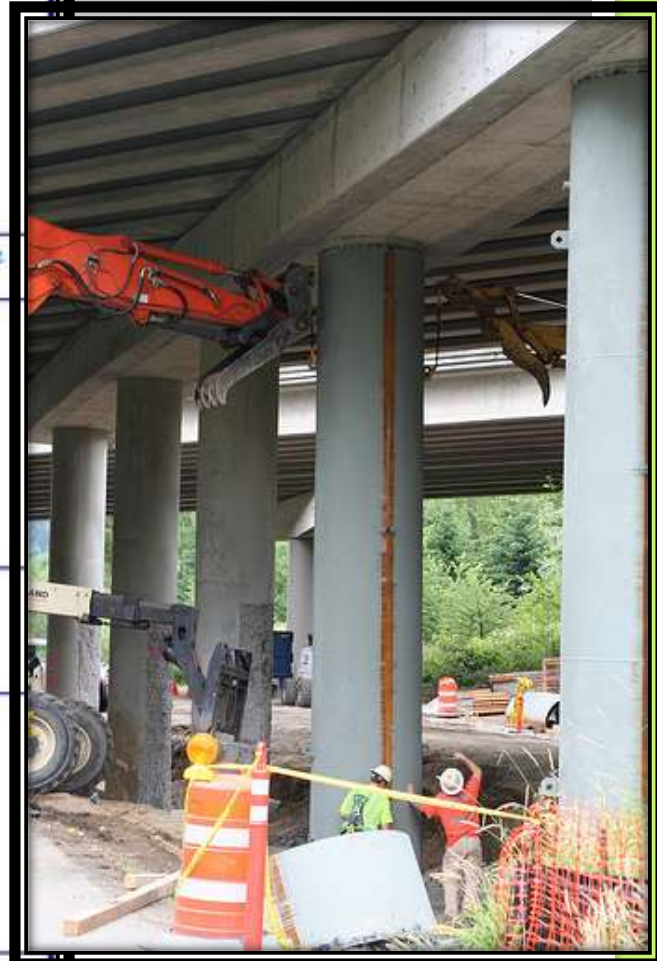
Step#1: Removing the concrete cover at the straps locations.
