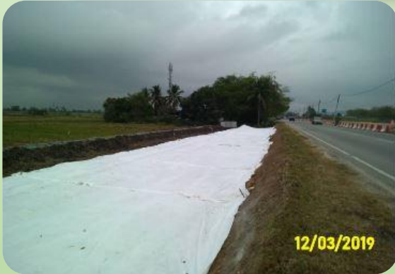
Laying of Geotextile
