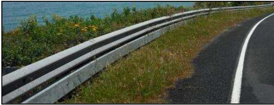
Figure 8.2: Photograph of Rub Rail Fitted To an Existing W-Beam (Source: Safe Direction)
