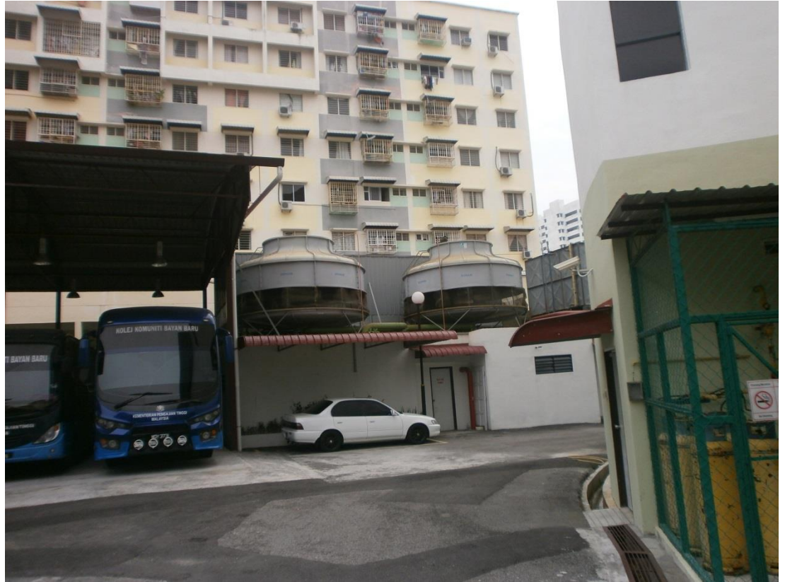
Figure 3.2 The picture of two cooling towers at the back of the building. A proposal will be made to remove them at the end of this report.
