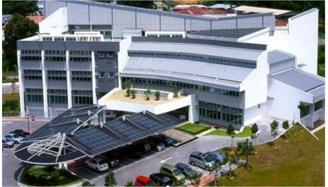
Figure 2.3 View of a zero-energy building building in Bangi, Selangor.
