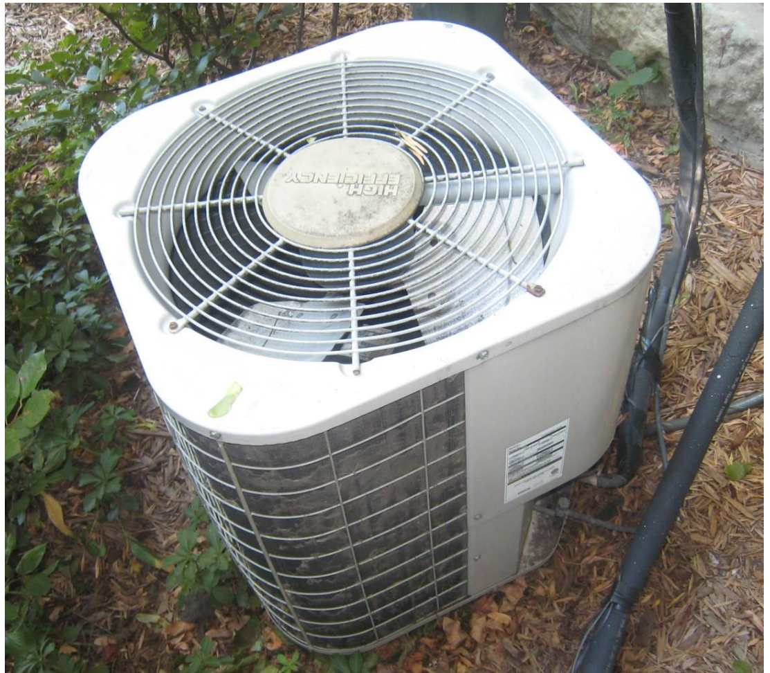
Figure 2.8 The compressor is located inside this outdoor unit
