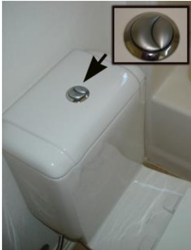
Figure 2.4 Dual flush water that lessen the water usage
