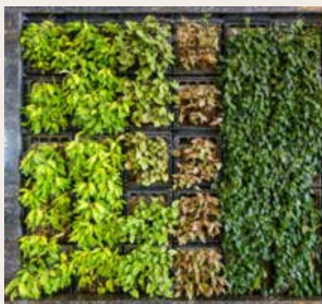
Figure 6: VGS using cassette system
