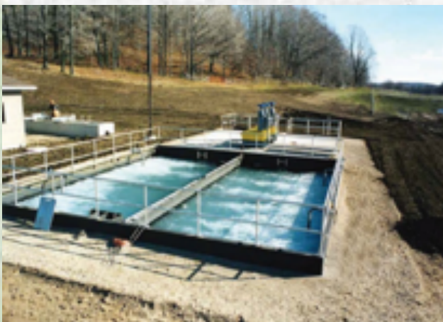
Figure 3: Extended Aeration Plant
