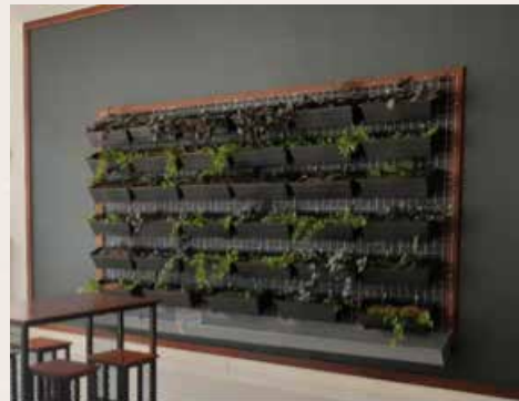
Figure 12: VGS-planter system installed on the wall of dining area, level 2 at Block A
