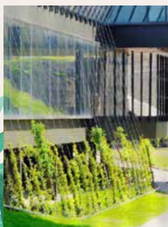
Figure 9: 'Green curtains' installed at building in Malaysia
