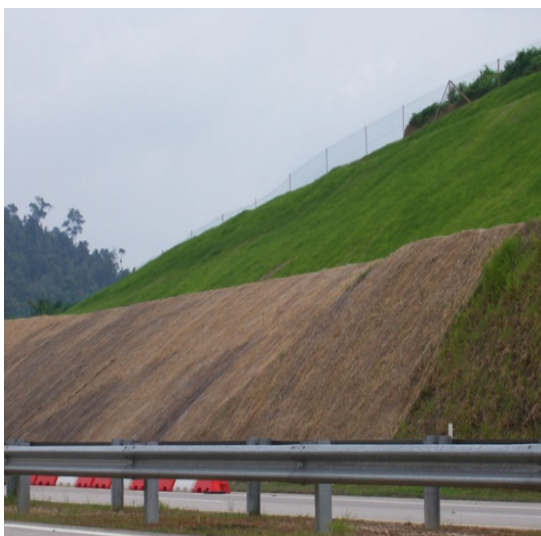
Figure 10: Application of Biodegradable Erosion Control Blanket Layer at Slope
