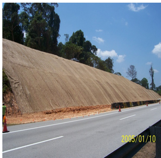
Figure 10: Application of Biodegradable Erosion Control Blanket Layer at Slope
