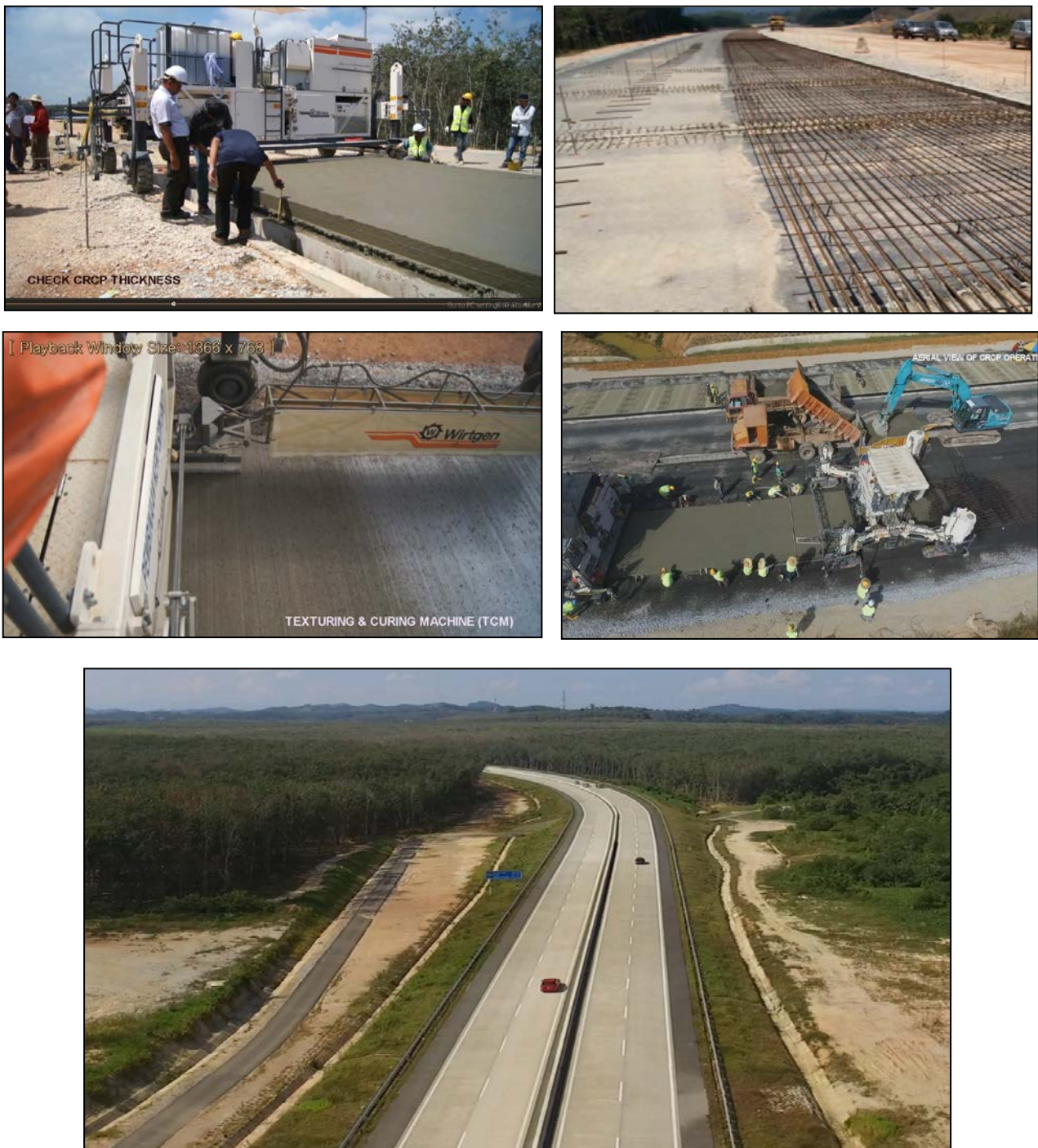
Figure 5: Photos taken from PAKEJ 3: GUA MUSANG, KELANTAN KE KG. RELONG, PAHANG -SEKSYEN 3H: FELDA TELANG KE KG. KECHUR whereby concrete pavement was adopted for this project.
