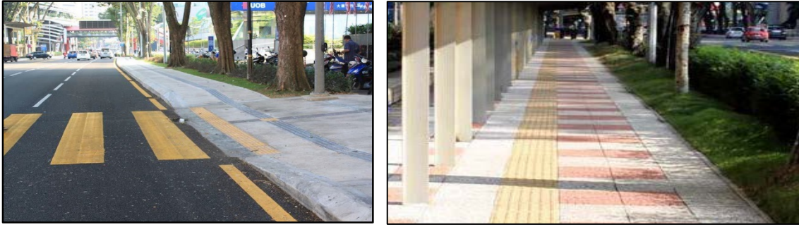
Figure 2: Example of Services for Disable Users: Ramp for Disabled Users at Zebra Crossing and Tactile on Pedestrian Walkway
