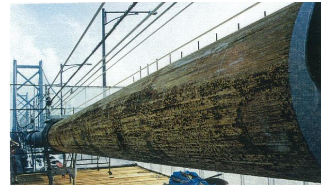
Corrosion of a main cable
