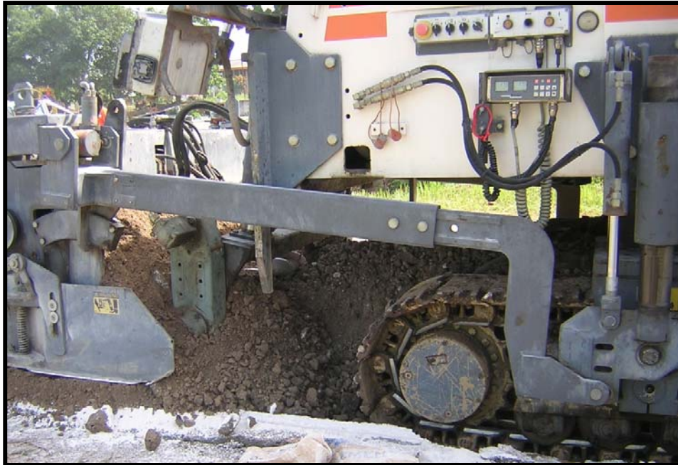
Figure 34: Reclamation of existing pavement for reuse
