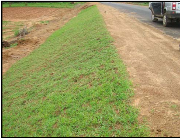
Figure 3 : Close turfing on earth surface
