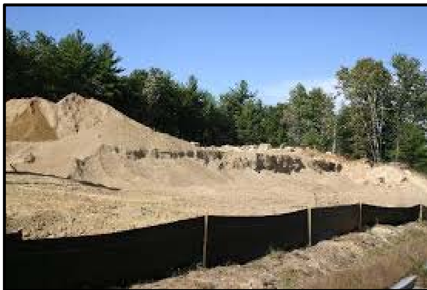
Figure 19 : Silt fence
