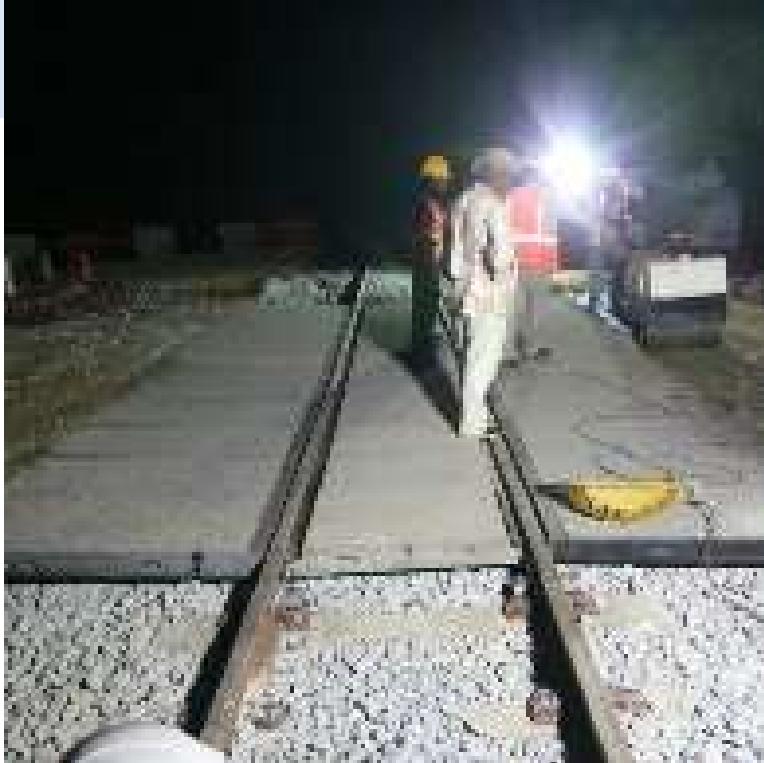
Final checking & inspection work by JKR & KTMB with contractor prior opening to traffic
