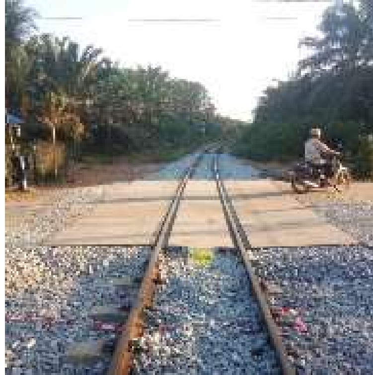
Routine checking & inspection work by JKR after opening for traffic
