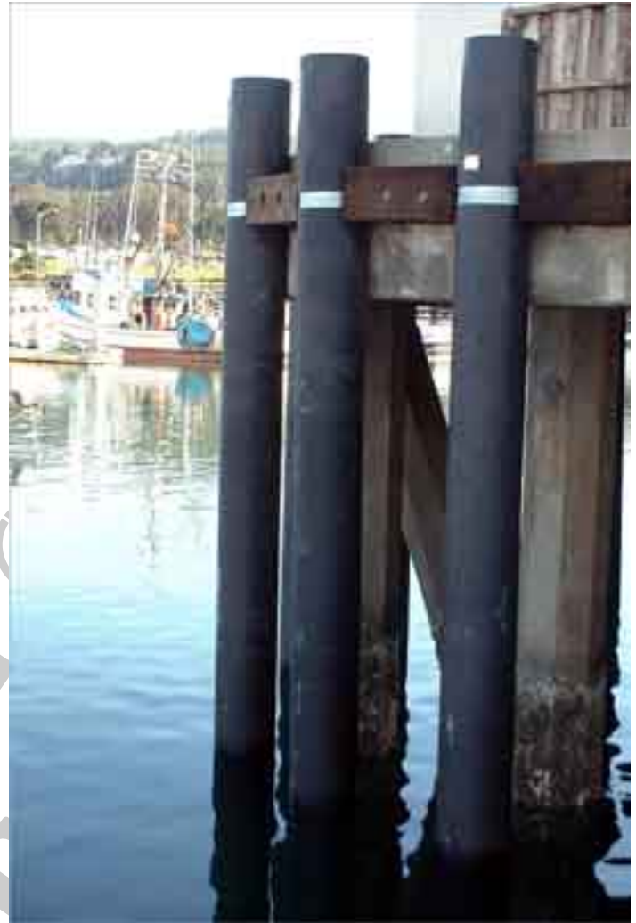
Figure 2-15 Plastic Composite Piling in Marine Application
