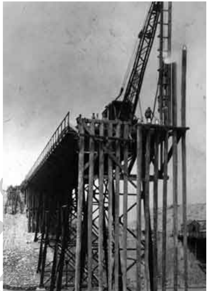
Figure 2-14 Timber Piling Driven for a Bridge
