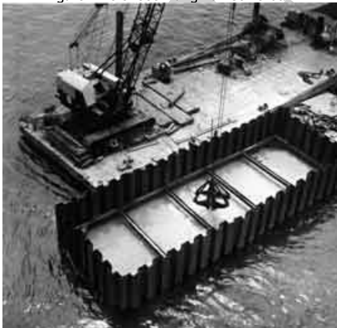
Figure 2-25 Sheet Piling Box Cofferdam
