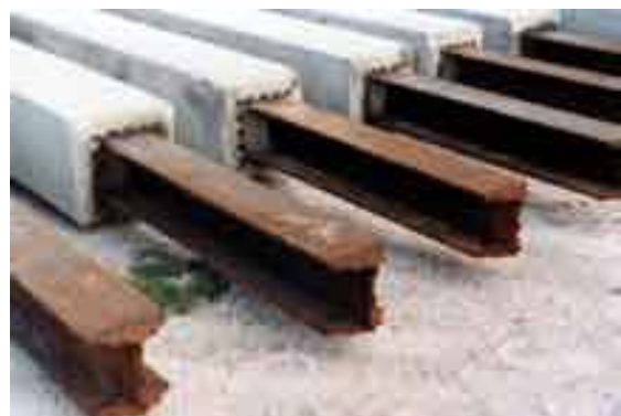
Figure 2-10 H-pile "Stinger" on Concrete Pile
