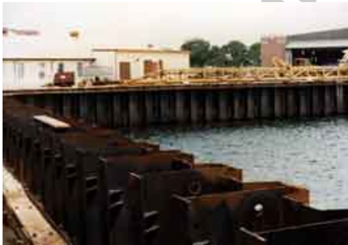
Figure 2-23 Master Pile Wall
