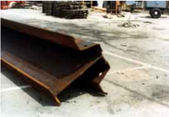
Figure 2-22 Master Pile Section
