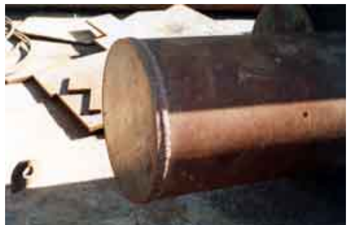
Figure 2-3 Closed End Pipe Piles
