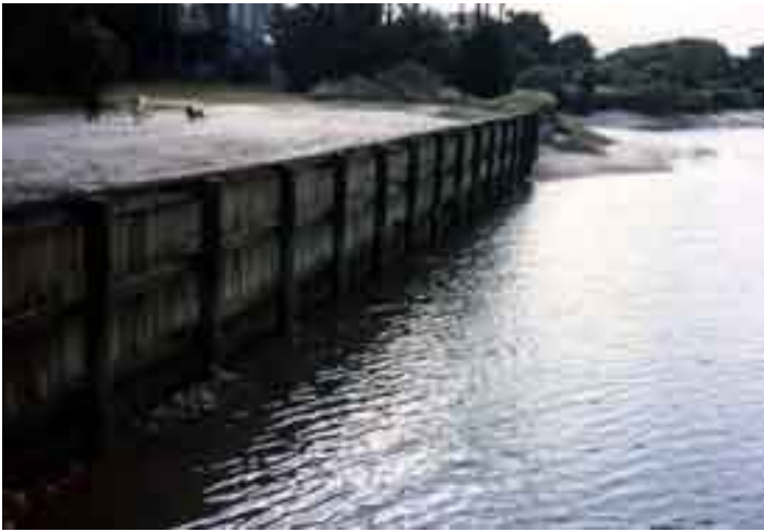
Figure 2-37 Completed Timber Bulkhead
