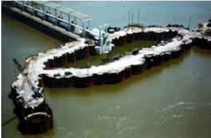
Figure 2-21 Cellular Cofferdam
