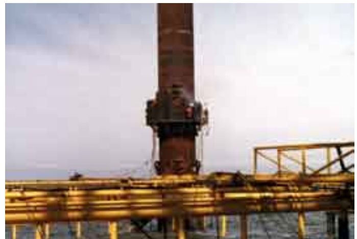
Figure 2-5 Welding an Add-On to Pipe Pile
