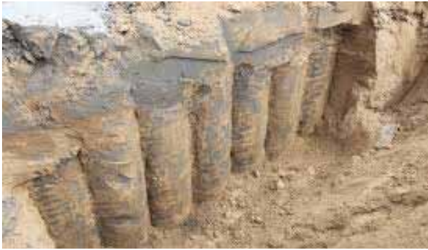
Rajah 2: Produk Akhir Deep Soil Mixing
