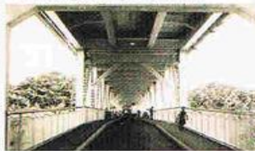
• Kota bridge in 1960s
