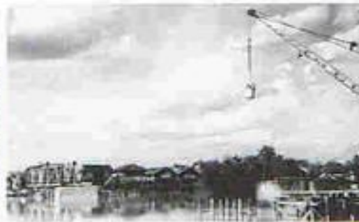
• Kota bridge during construction.
