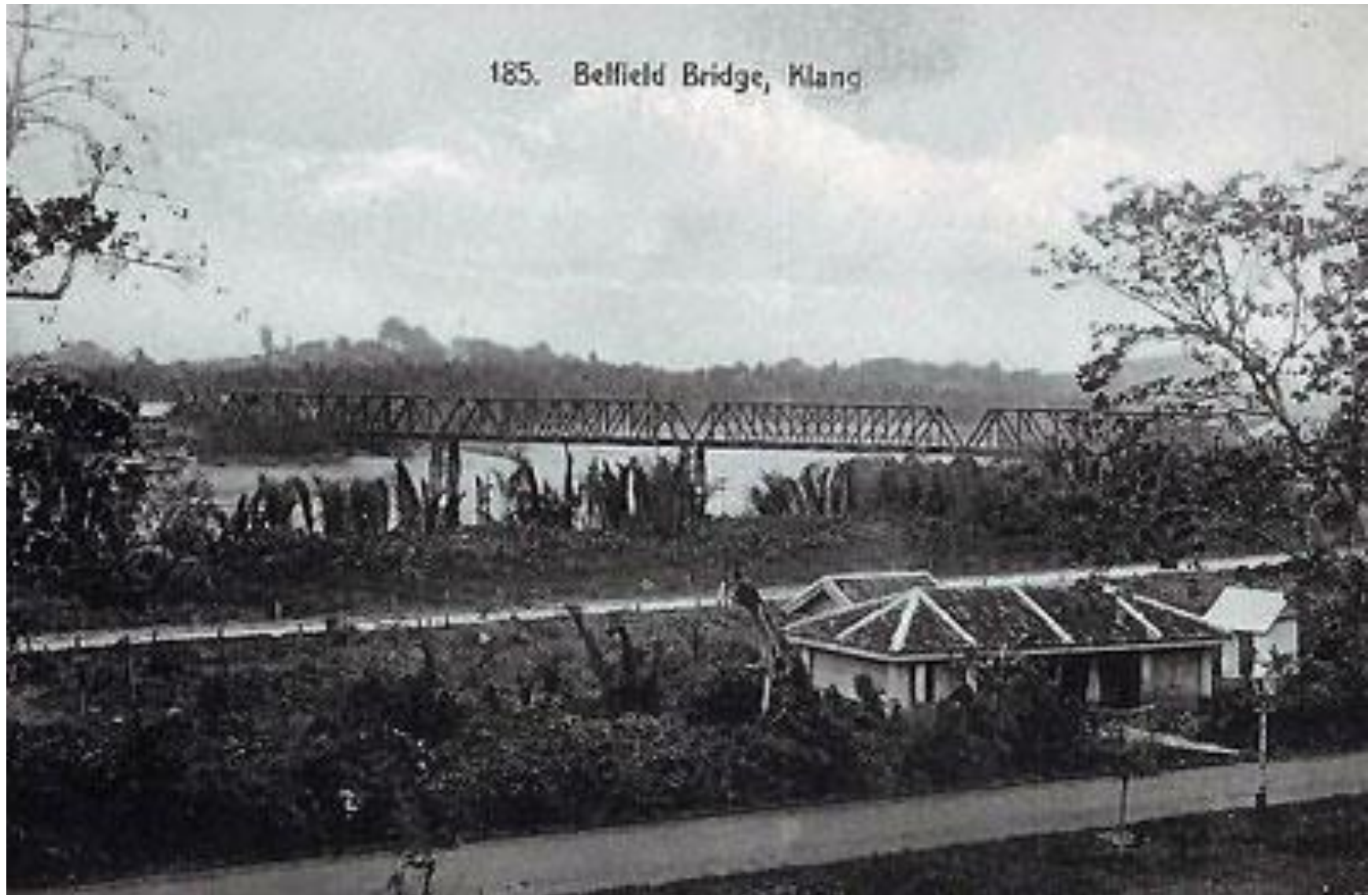
Belfield Bridge Klang
