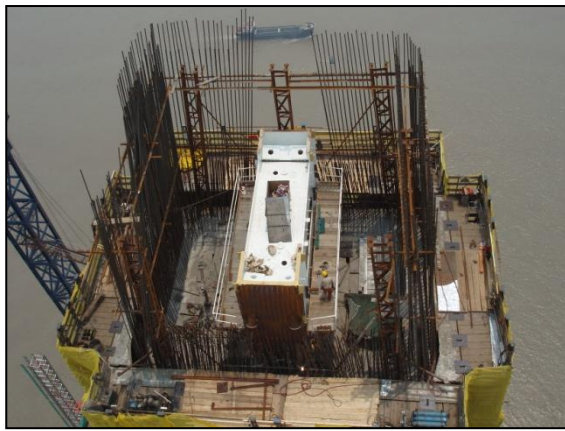
Figure 20 –Upper Tower Stay Anchor Box Installation
