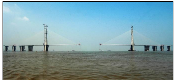
Figure 18 – Sutong Bridge Main Span Erection
