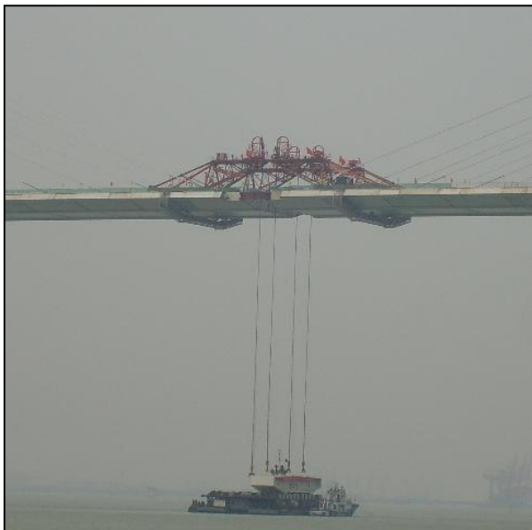
Figure 24 – Main Span Closure
