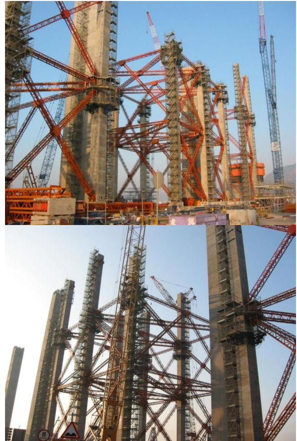
Figure 8 – Backspan Falsework
