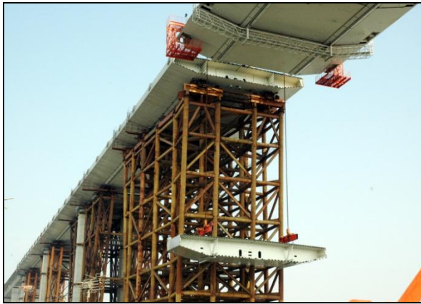
Figure 23 – Backspan Closure
