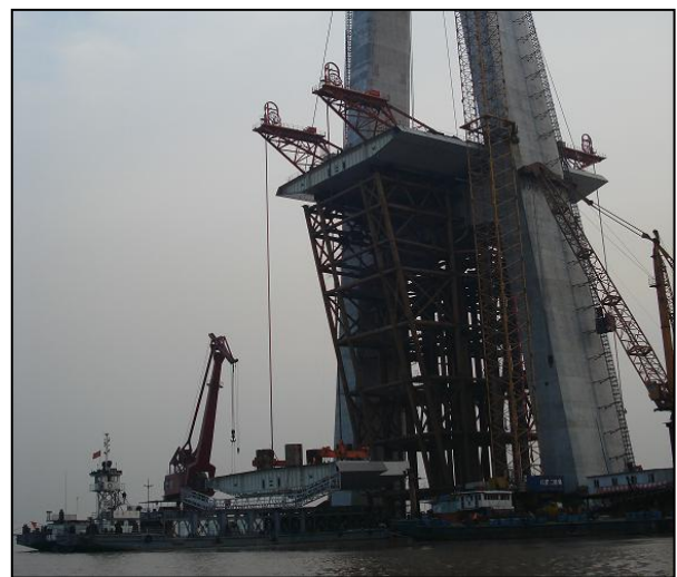
Figure 22 – Cantilevered Segment Erection
