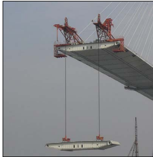
Figure 25 – Segment Erection Cycle
