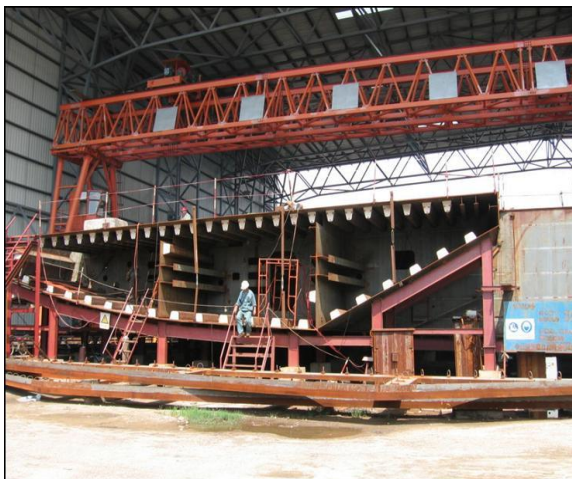
Figure 11 – Deck Segment Assembly
