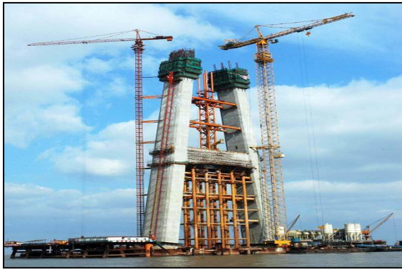
Figure 19 – Tower Shaft Construction
