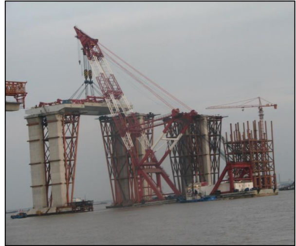
Figure 21 – Backspan Segment Erection
