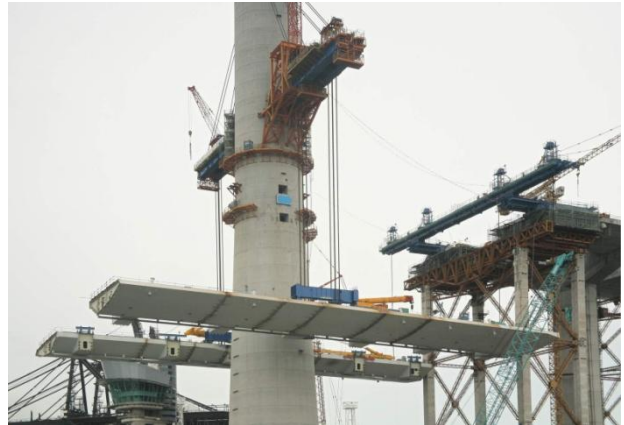
Figure 12 – Heavy Lift Operation
