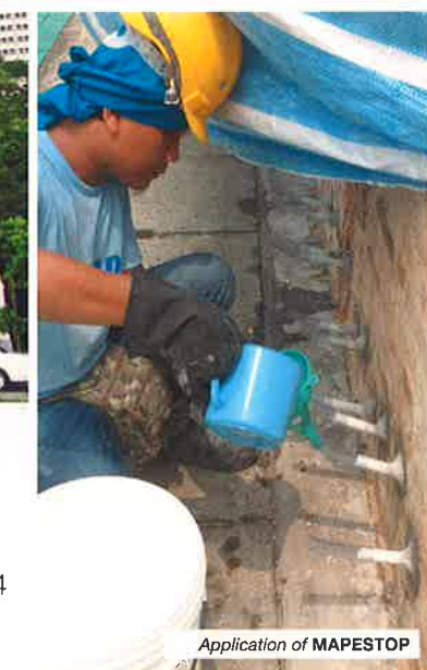
Crack repairs with EPOJET LV
