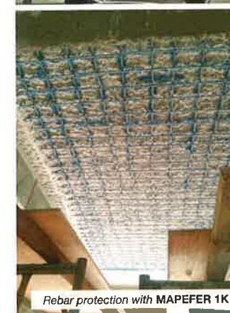
Spray application of MAPEGROUT THIXOTROPIC
