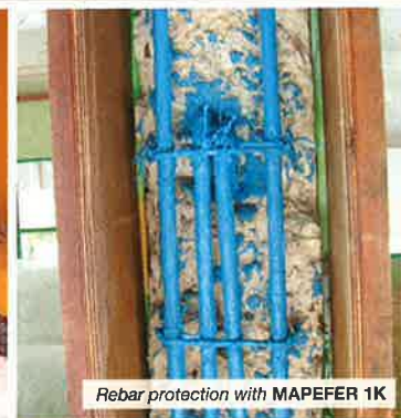
Spalled concrete at column
