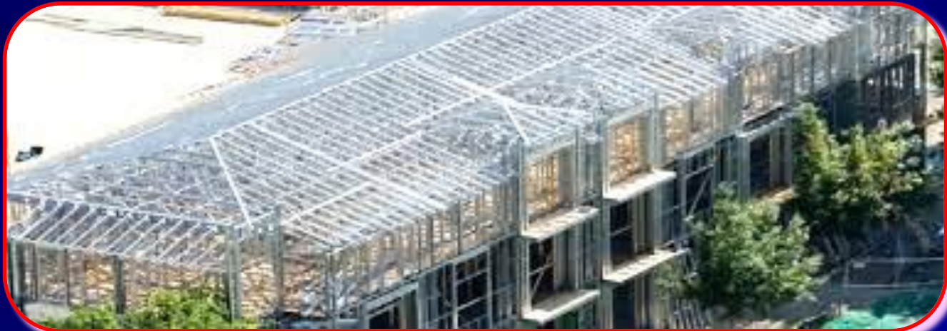
Cold-formed Steel Roof Trusses
