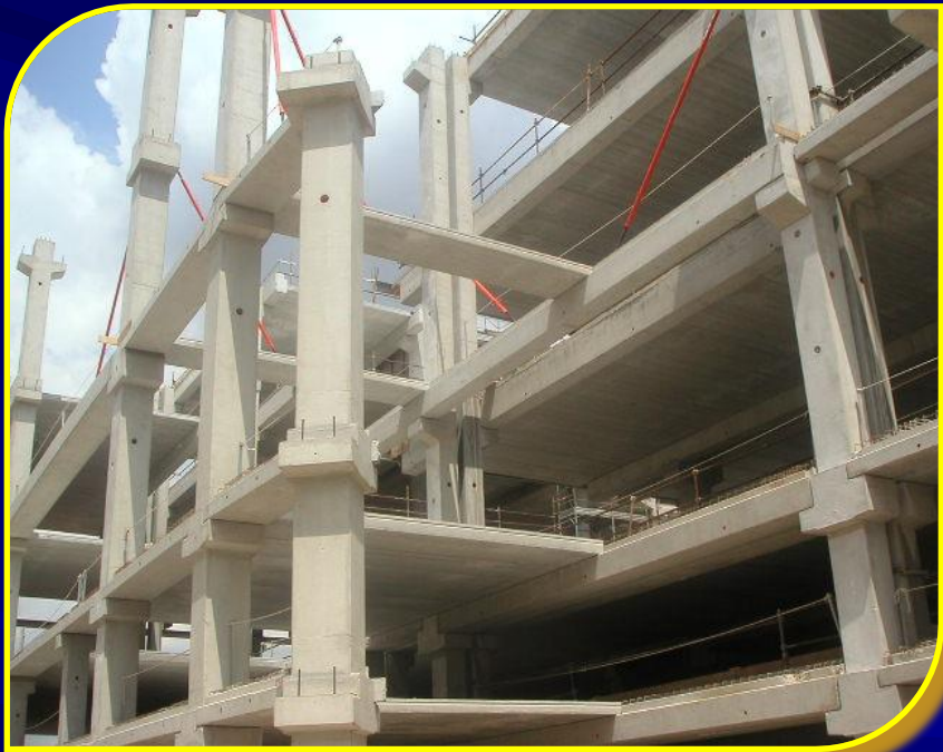
Precast Concrete Structure
