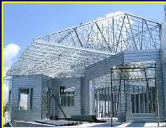
Cold-formed Steel Roof Trusses
