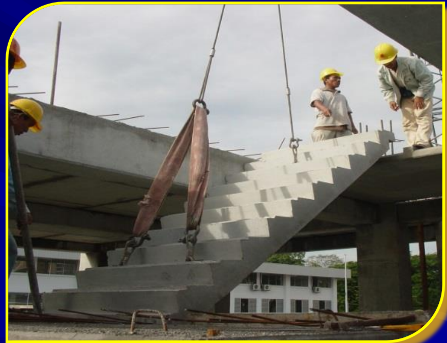
Precast Concrete Staircase
