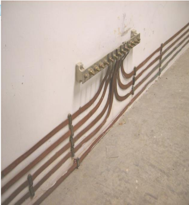
Centralized Earthing
