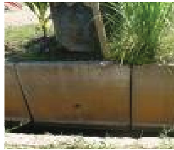
Gap antara joints > 6mm.
