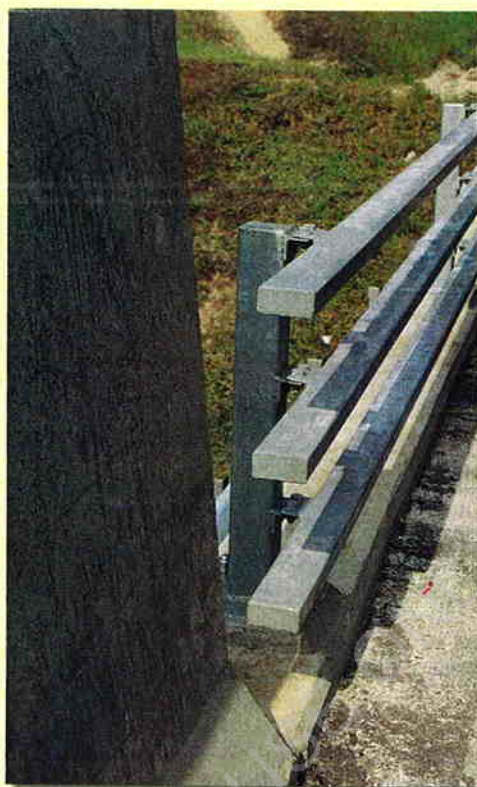
Photo 6 Misalignment of the concrete bridge barrier with the adjacent bridge railing and the 'spearing' projections of the rails result in a very unsafe arrangement.
