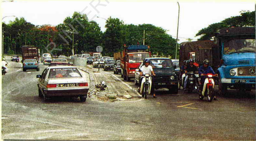
Picture 19 : Signal post located too closed to the median nose Note that the signal pole in the narrow media has been knocked down.
