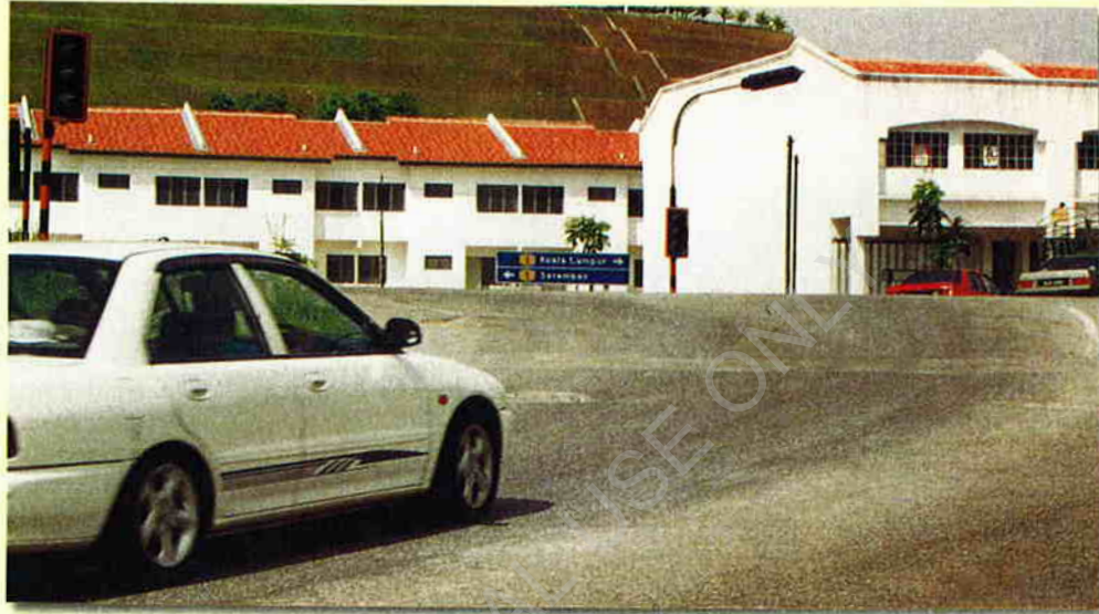
Picture 18 : Lack of channelisation in the side road and visibility of the highway.
