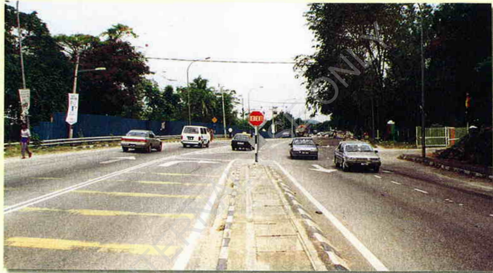
Picture 22 : A 'trap' lane in High School Entrance. Note also the incorrect use of the 'Berhenti' (STOP) Sign.
