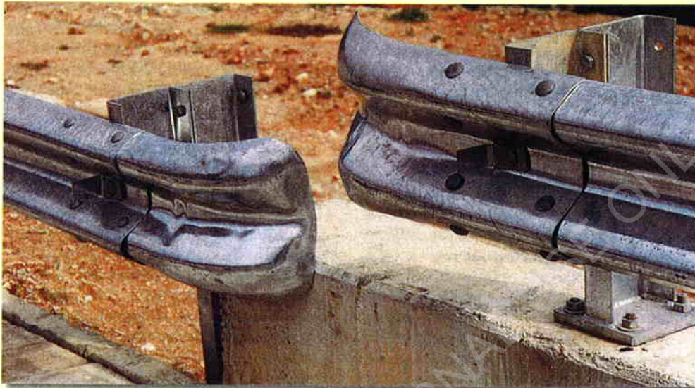
An improper guardrail to bridge rail connection like this can be corrected at the construction stage.
