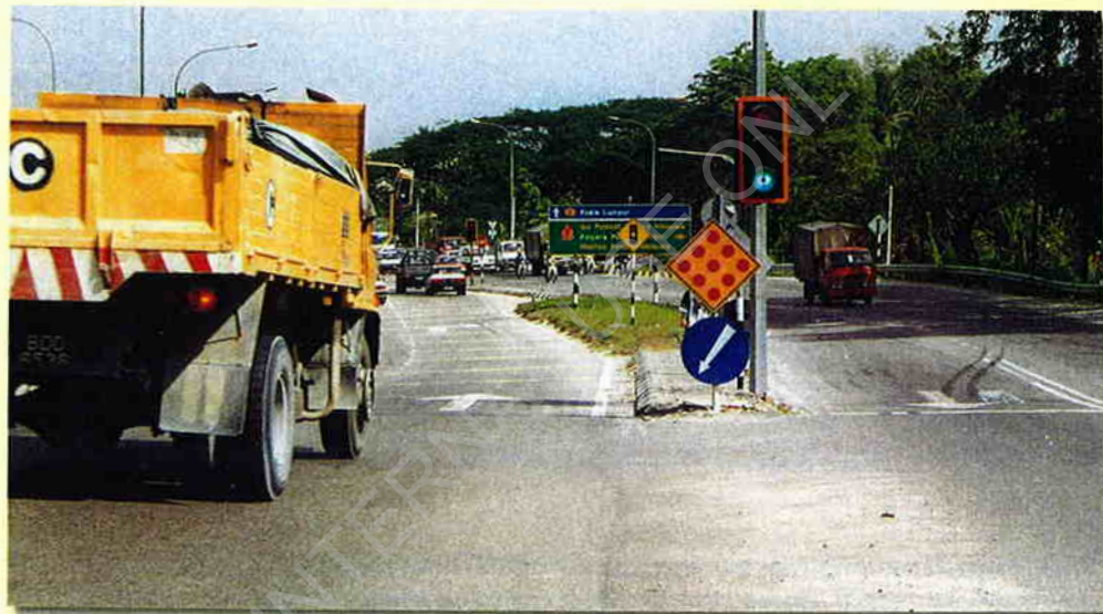
Picture 14 : Street lights and traffic sign posts all mounted very close to the road edge.
