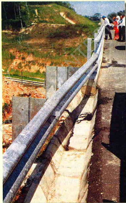
Photo 8 Another case of inadequate guardrail to bridge rail connection. The lack of stiffness and strength in the last two sections of guardrail leaves a high probability of a heavy impact going through the guardrail onto the railway below. Note also the deep roadside drain in front of the guardrail, which may alter the way the guardrail performs.
