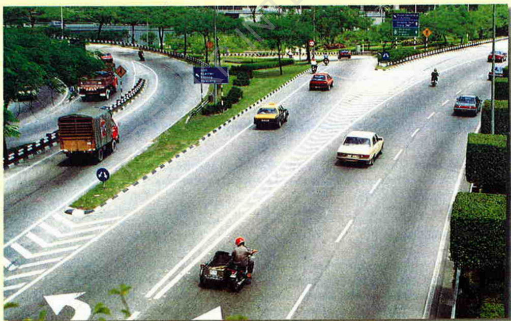
At a complex exit arrangement like this, is this standard of direction signing adequate? The signs here lack prominence and have poor legibility.
