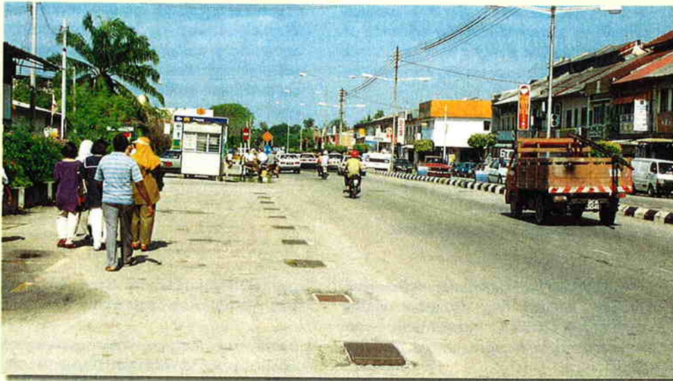
The traffic signals here lack visibility and prominence, and some signal heads are hidden by traffic signs
