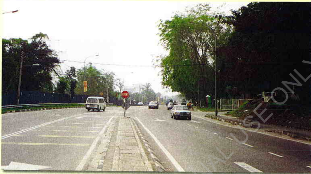
Picture 24 : Poor visibility for right turners into the High School due to crest hill.
