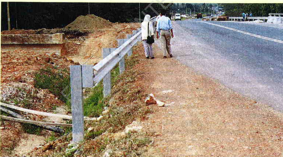
This bridge approach guardrail runs off the verge onto the embankment slope, resulting in inadequate ground support for the posts.
