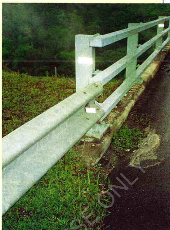
Inappropriate connection and transition of the approach guardrail to the bridge rail system in these photo's will have serious consequences for an impacting vehicle.
