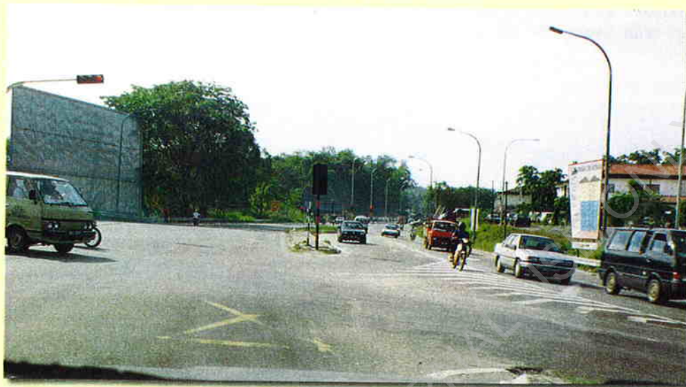
Picture 16 : 'Seagull' type treatment involves a 'trap' lane for the right turners.
