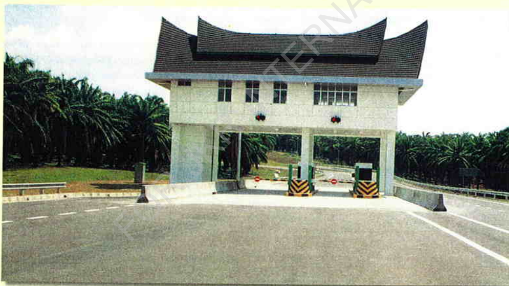
Photo 7 The ends of the New Jersey barrier past the Toll Plaza pose considerable hazard in an area where unpredictable traffic movements often occur. The 'high speed approach (beyond the Toll Booths in this picture) particularly justifies treatment with an appropriate 'crash cushion'.
