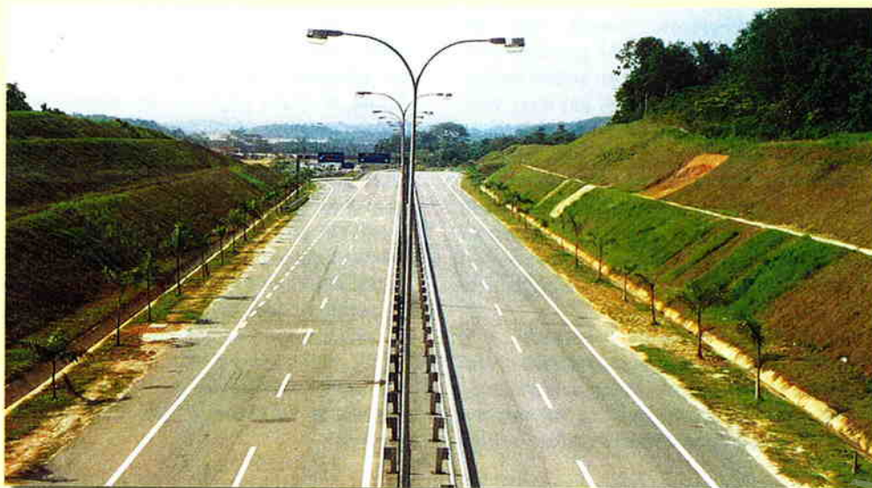
Photo 14 In view of the high speed environment of the Expressway, is it appropriate to plant the palm trees so close to the edge of the roadway? Note that there is ample space beyond the side drains and along the toe of the cut slope to plant trees, where they will be less of a hazard to motorists and motorists less of a hazard to the trees.
