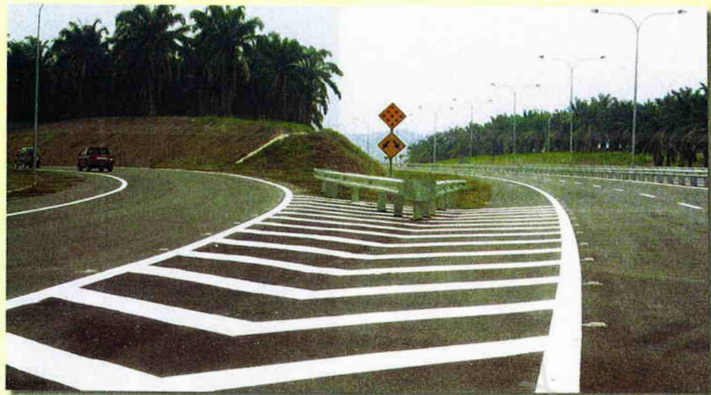
Photo 4 Unnecessary guardrail located in the hazardous Exit 'gore area'
