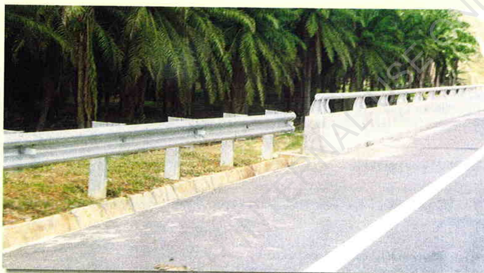
Photo 2 Failure to connect the approach guardrail to the bridge barrier system. Note that there is no anchorage provided at the end of the guardrail.
