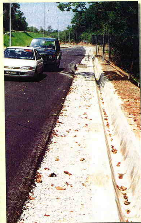
Photo 9 The deep roadside drain here is very close to the traffic lanes and poses a serious hazard especially for motorcycle riders. The embankment height and slope also increase the severity of 'run-off' accidents. Note also the concrete foundation marking the position of a proposed traffic signal pole right on the edge of the pavement with no clearance or protection on this relatively high speed approach.
