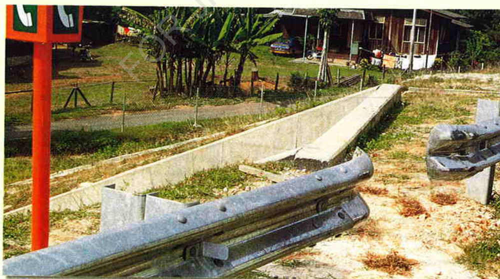
Photo 3 Unsafe gaps in the guardrail at the emergency telephones.
