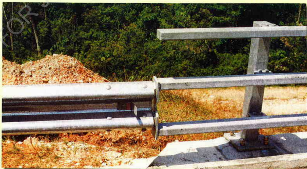
Photo 5 Unsatisfactory joining of the approach guardrail to the bridge railing system: No transition of rigidity of the guardrail as it approaches the bridge. Note also the 'spearing' danger created by allowing the bridge rails to extend beyond the end post of the bridge.
