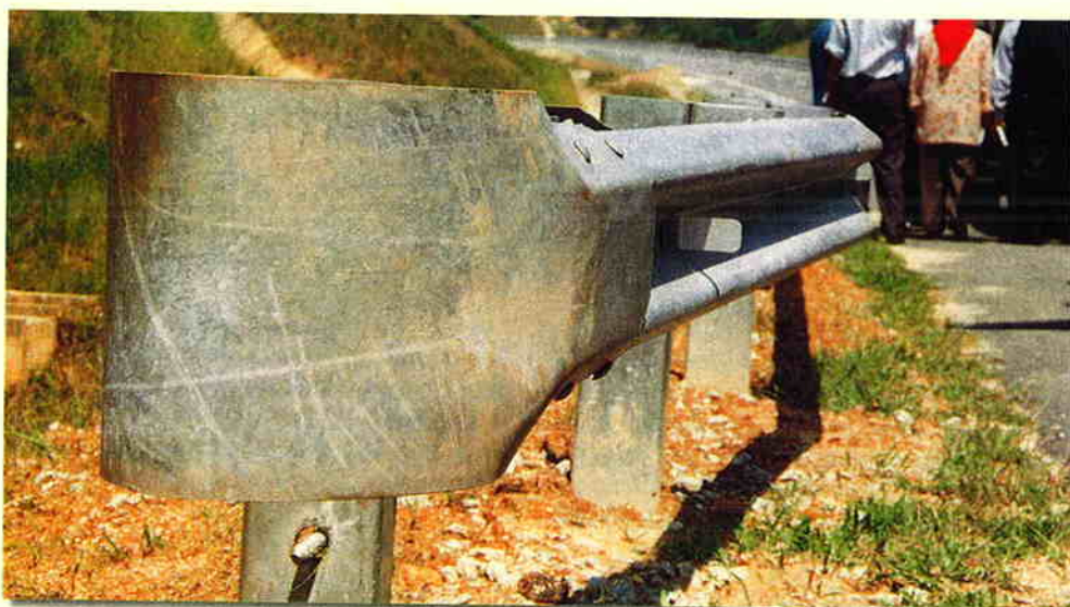
Photo 1 Improper guardrail terminal. Note the absence of nut and washer on the end of the anchor rod and the excessive height of the anchor point above the ground.
