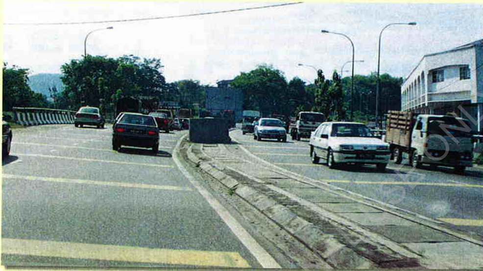
Picture 20 : Large concrete buttress constructed in the median.
