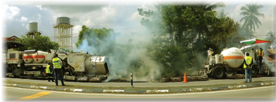
Hot In-Place Recycling.
