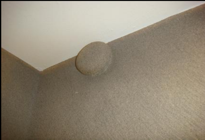
Bell system ditutup
