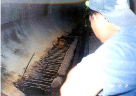
Failure at the bottom of culvert
