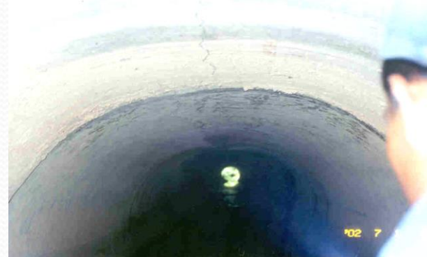
Crack and water ponding on the inside of culvert
