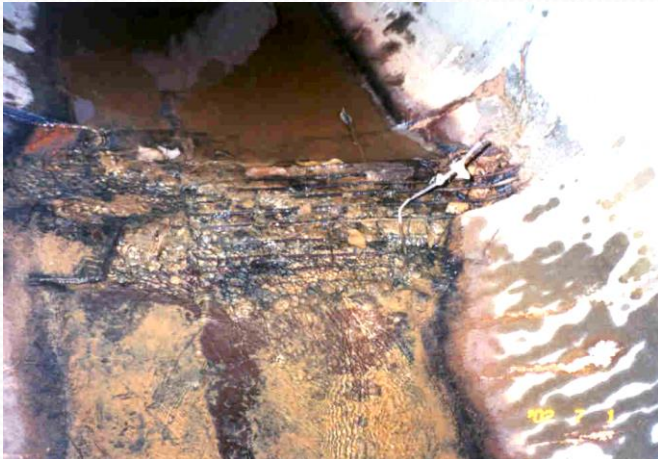
Failure at the bottom of culvert
