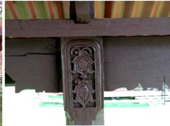
Figure 6.15: The carvings in the original colour and actual position of the Serambi's beam (facing inside) (left). The carvings were painted in timber colour and in the wrong position (facing outside) (right)
