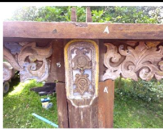
Figure 6.15: The carvings in the original colour and actual position of the Serambi's beam (facing inside) (left). The carvings were painted in timber colour and in the wrong position (facing outside) (right)
