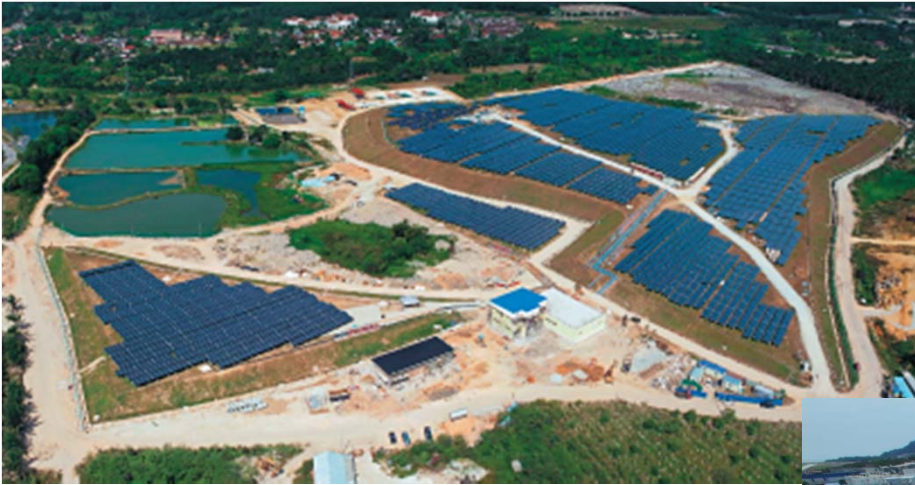
8 MWp at Cypark, Pajam
