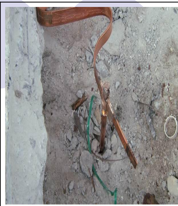
Example of Earthing System
