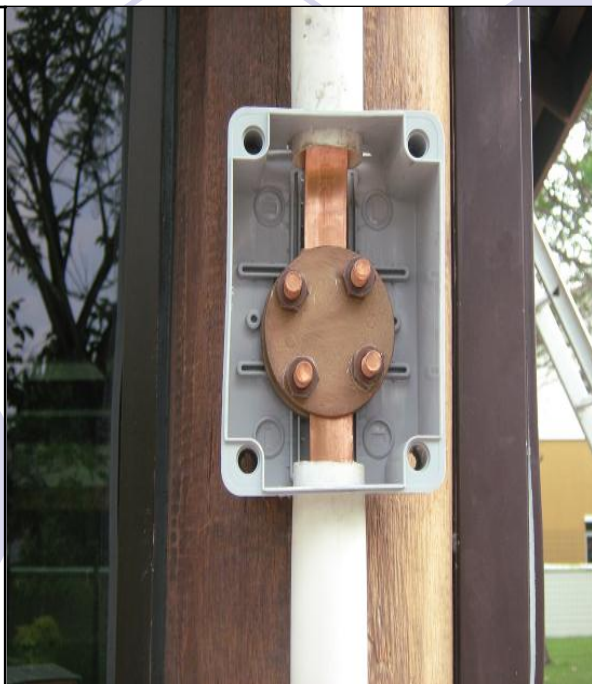
Example of Down Conductor System
