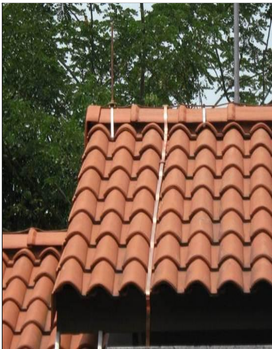
Example of Air Termination System
