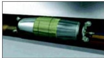
STEP 5: Air pressure is used to inflate the packer. The resin impregnated fibre glass is pressed over the defect and held in place until the resin cures
