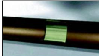
STEP 6: The packer is deflated and removed from the pipe. The section repair has now fully sealed the defect
