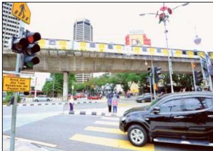
FIGURE 5.2: THERMOPLASTIC COLORED ZEBRA CROSSING AT STOP INTERSECTIONS
