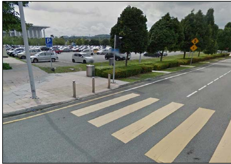
FIGURE 5.1: INTERLOCKING BLOCK LEADING TO PEDESTRIAN CROSSING
