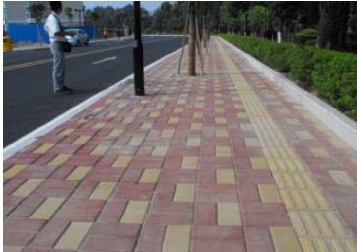
FIGURE 5.3: TACTILE INTERLOCKING AND GUIDING BLOCK FOR THE VISUALLY IMPAIRED
