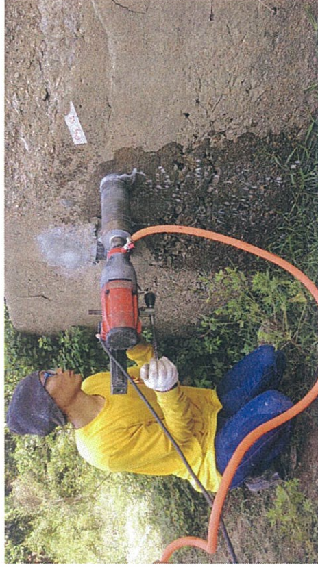
Concrete Core Extraction at Pier 5.
