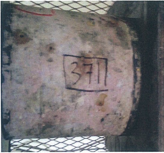
The prepared Concrete Core extracted from Pier 5.
