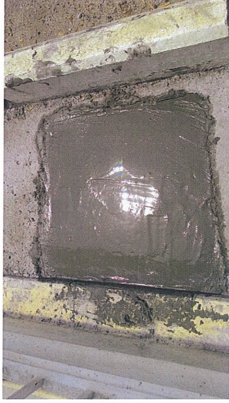
Picture 3 - Reinstatement Works to Deck Slab.
