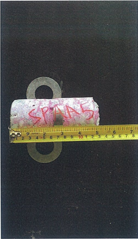
Picture 5 - Carbonation Test to sample from Span 5 Slab.
