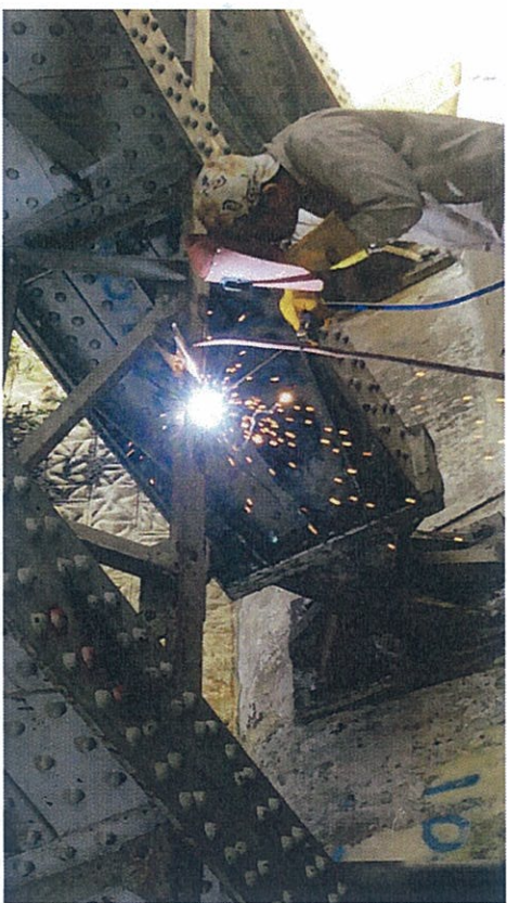
Picture 2 - Reinstatement of cut section for TS1 at Span 7.
