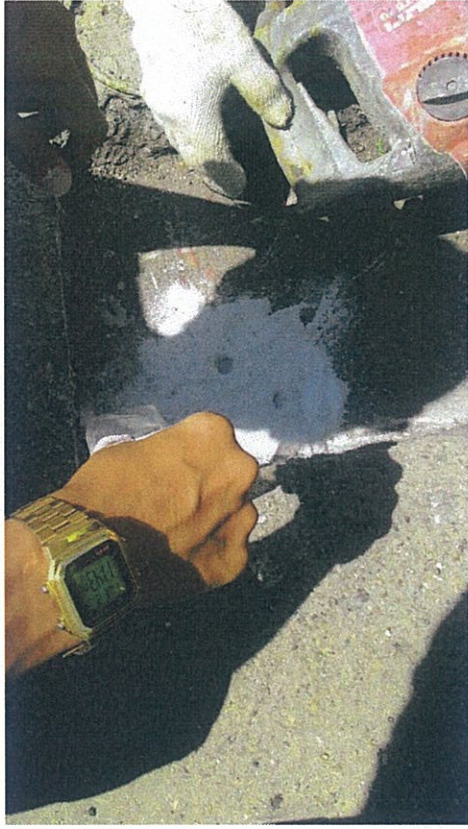
Picture 1 - Dust Sampling at Deck Slab.
