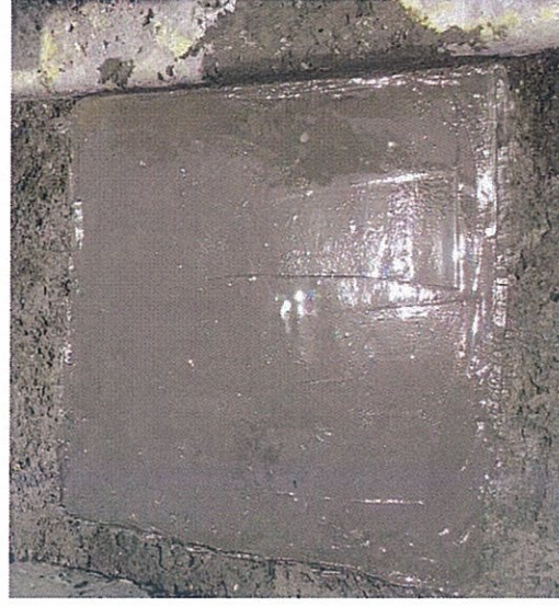
Picture 4 - Reinstatement Works to Deck Slab.
