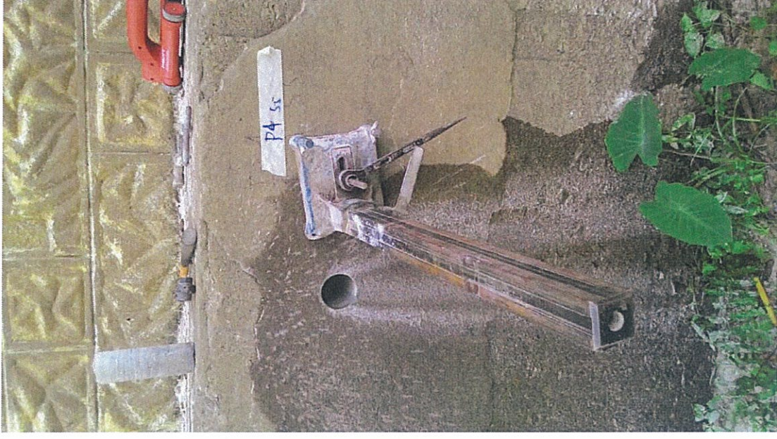
Picture 8 - Core Extraction at Pier 4.
