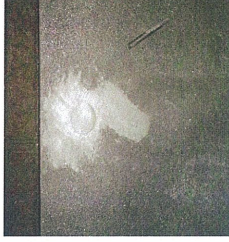
Patching Works at Pier 1.
