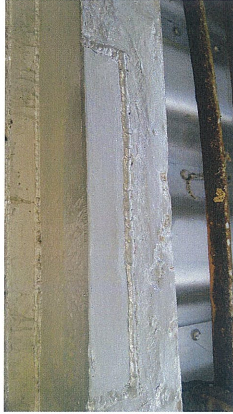
Picture 8 - Painting to the reinstated cut section at Span 7.
