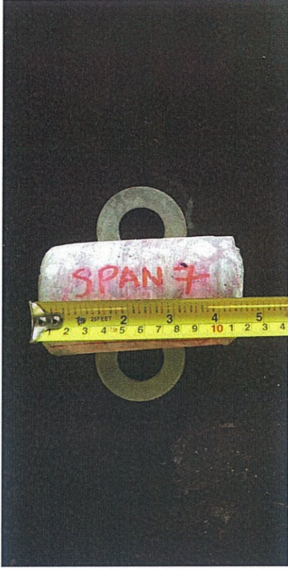
Picture 7 - Carbonation Test to sample from Span 7 Slab.
