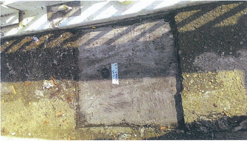
Picture 3 - Core Extraction at Span 3 Slab.
