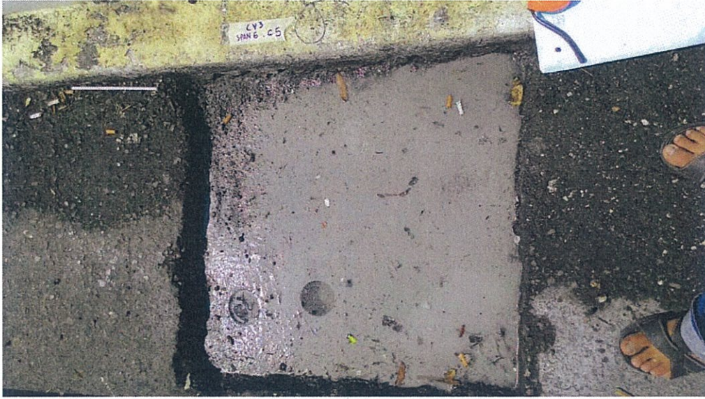
Picture 5 - Core Extraction at Span 6 Slab.
