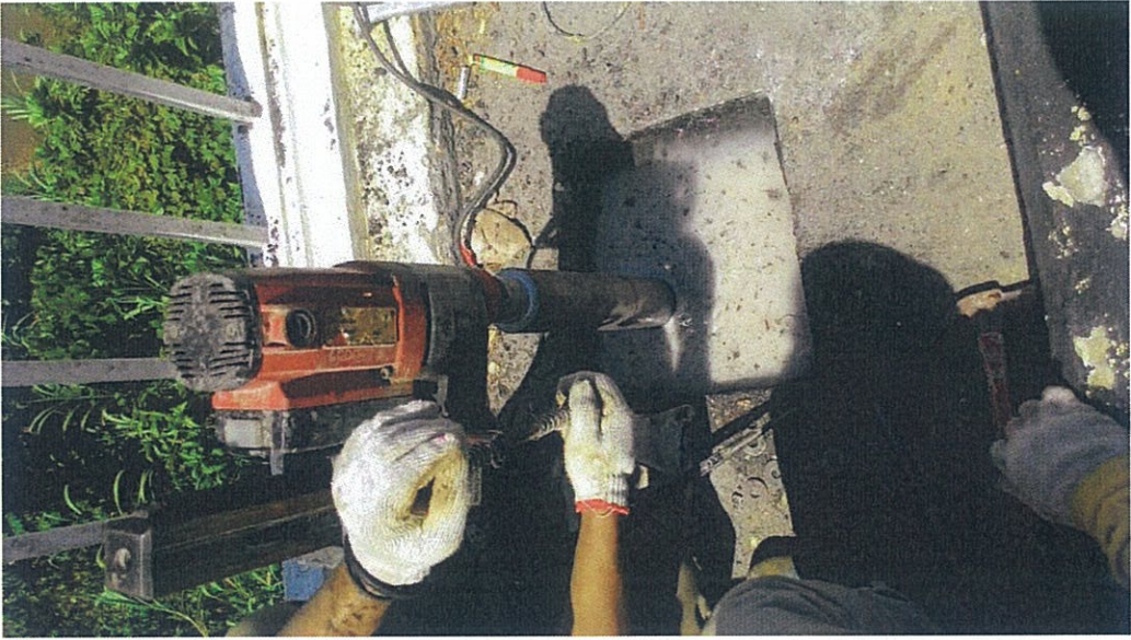
Picture 1 - Core Extraction at Span 1 Slab.
