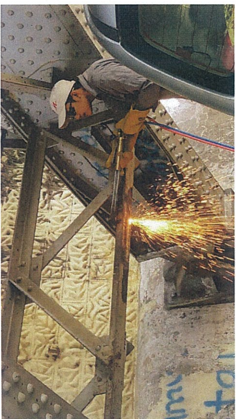
Picture 1 - Steel Extraction for TS1 at Span 7.
