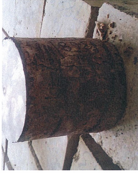
The crushed Concrete Core extracted from Abutment 1.
