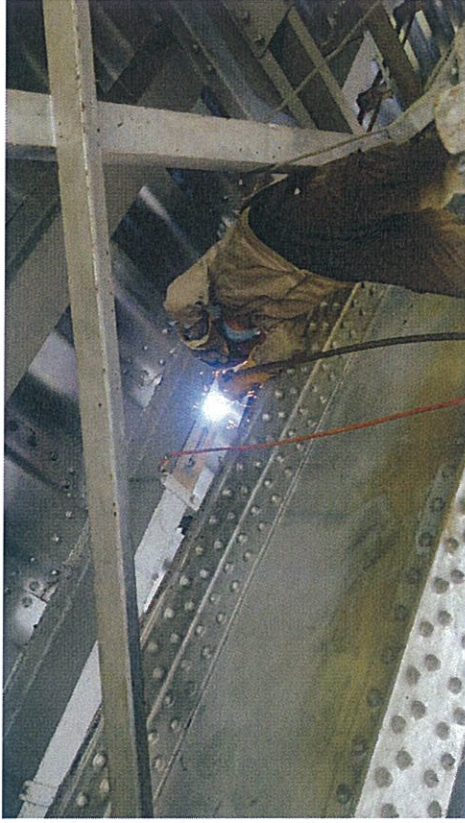
Picture 7 - Reinstatement of cut section for TS3 at Span 7.
