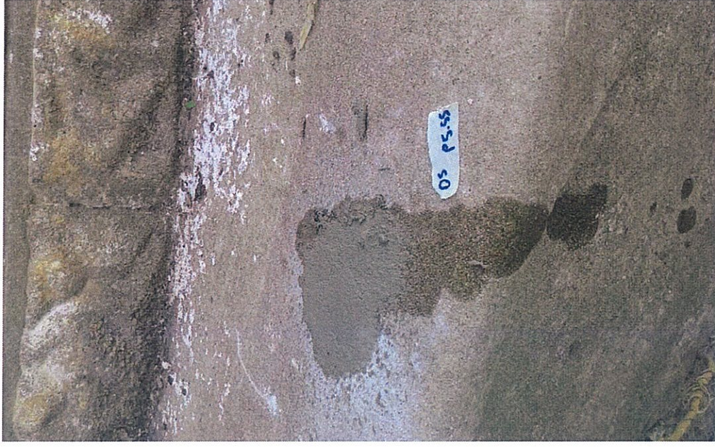
Picture 7 - Reinstatement Works to Deck Slab.
