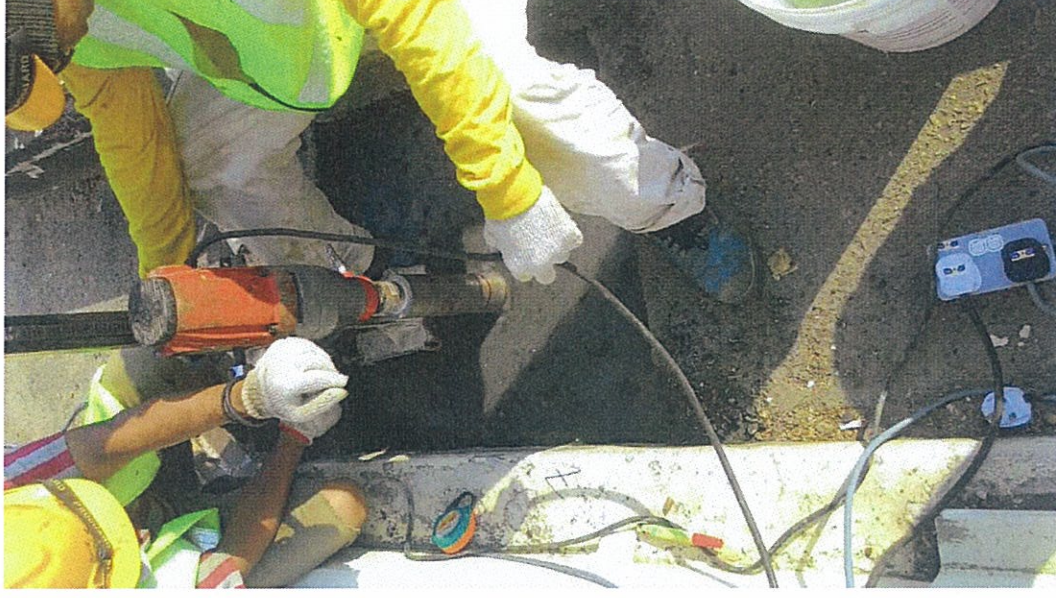
Picture 4 - Core Extraction at Span 5 Slab.
