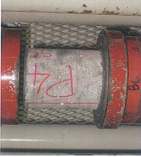
The prepared Concrete Core extracted from Pier 4.
