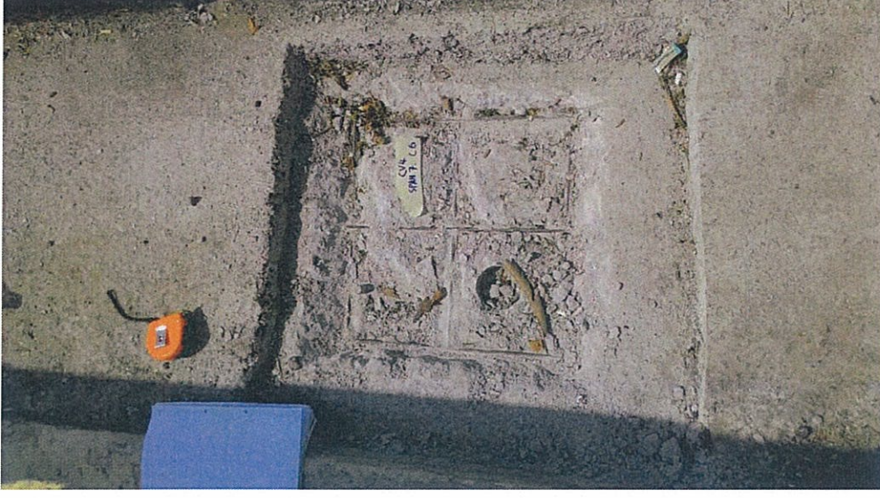
Picture 6 - Core Extraction at Span 7 Slab.
