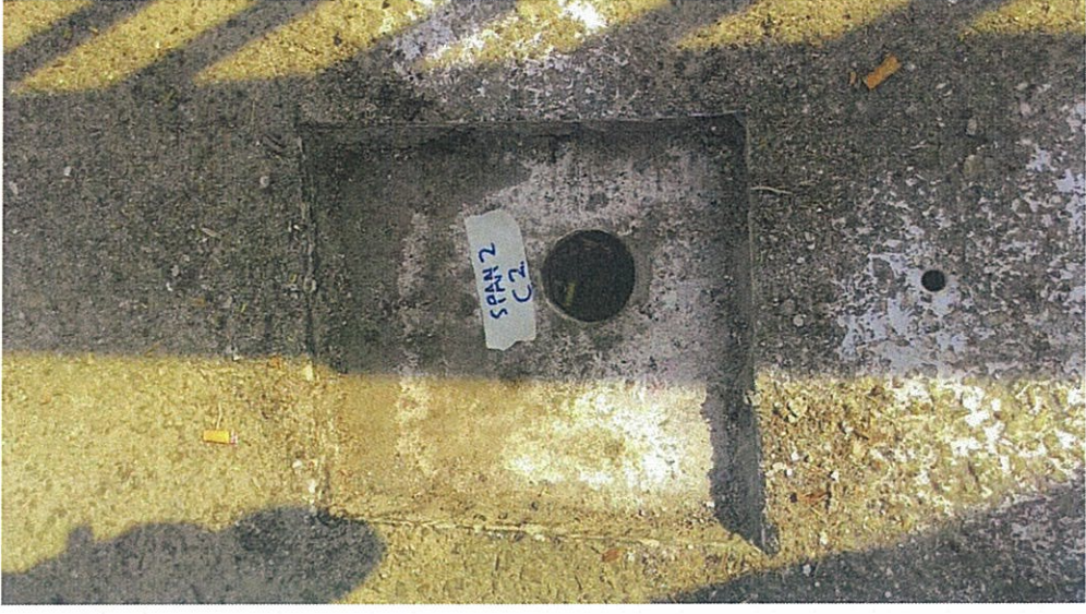
Picture 2 - Core Extraction at Span 2 Slab.
