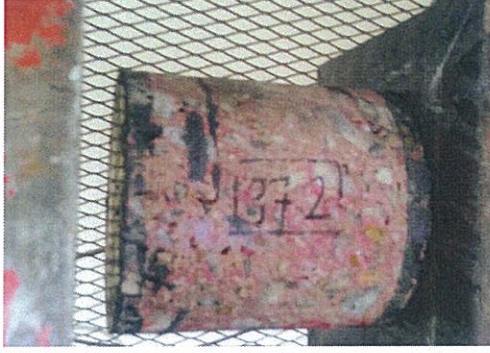
The prepared Concrete Core extracted from Pier 6.
