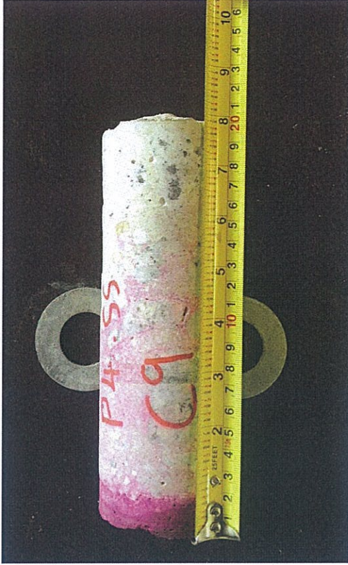
Picture 11 - Carbonation Test to sample from Pier 4.
