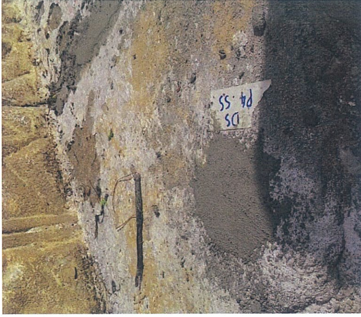
Picture 8 - Reinstatement Works to Deck Slab.
