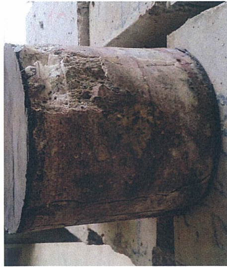
The crushed Concrete Core extracted from Pier 1.
