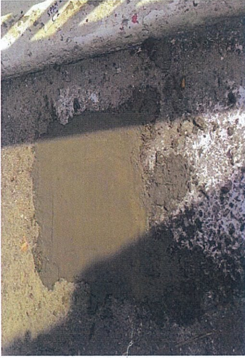
Picture 5 - Reinstatement Works to Deck Slab.
