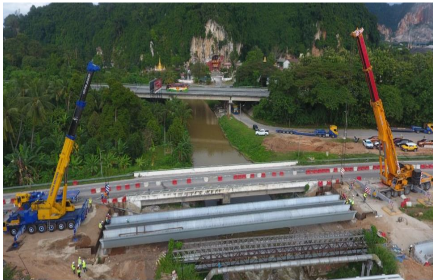
Figure 12: Photos taken from the project Sungai Rai Bridge, Perak whereby UHPC U-Beam was adopted for this project. Due to the characteristic of UHPC, longer span can be achieved (above 40m in length) and this provided the option to avoid the design of river pier. This will reduce the impact to the environment and also less obstruction to the river during the construction stage.
