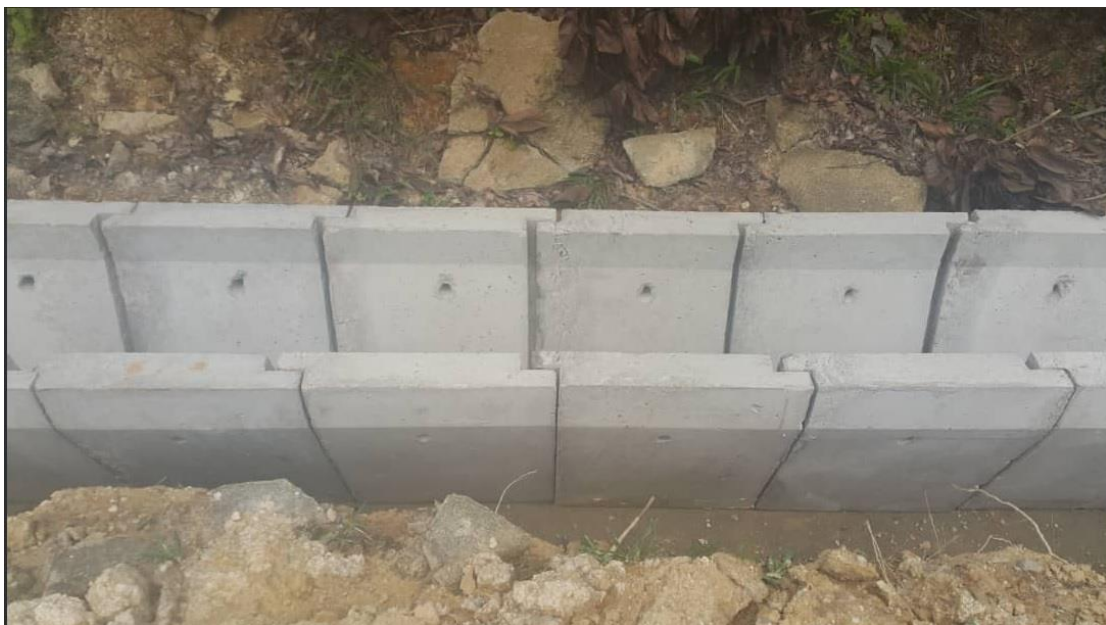
Figure 13: Photos taken from project at Jalan Bongkok, Bera whereby Tongue and Groove Shaped Concrete Drain was adopted for this project.
