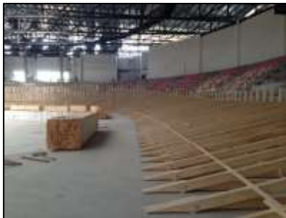
Installation for Under Carriage structure for Timber Track
