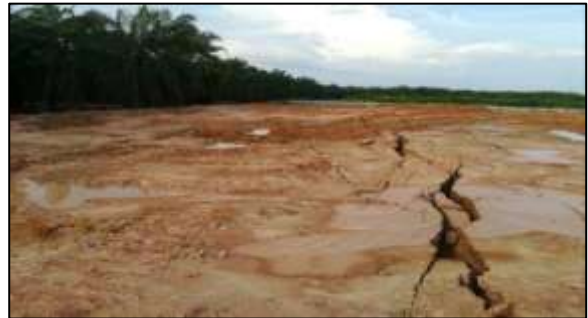
Rajah 4: Surface Tension Crack selepas Surcharge dibuat
