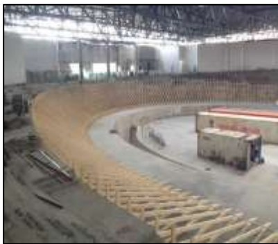
Installation for Under Carriage structure for Timber Track
