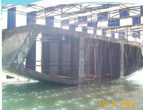
Curing of segment with automatic sprinkling system
