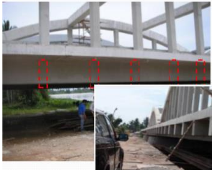
Transverse beam not constructed below walk way slab (Not following construction drawing)
