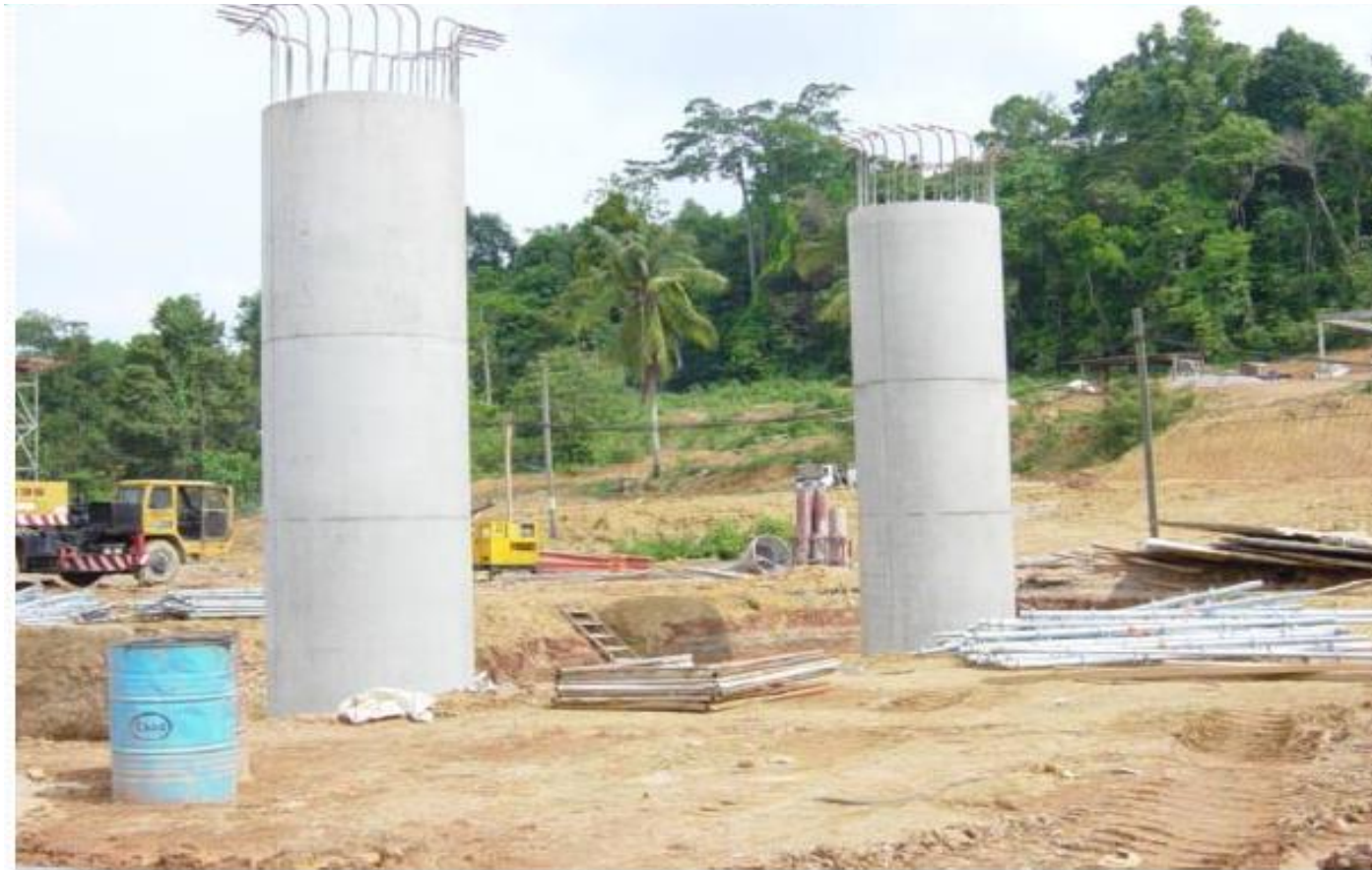
Piers: Good concrete finishing
