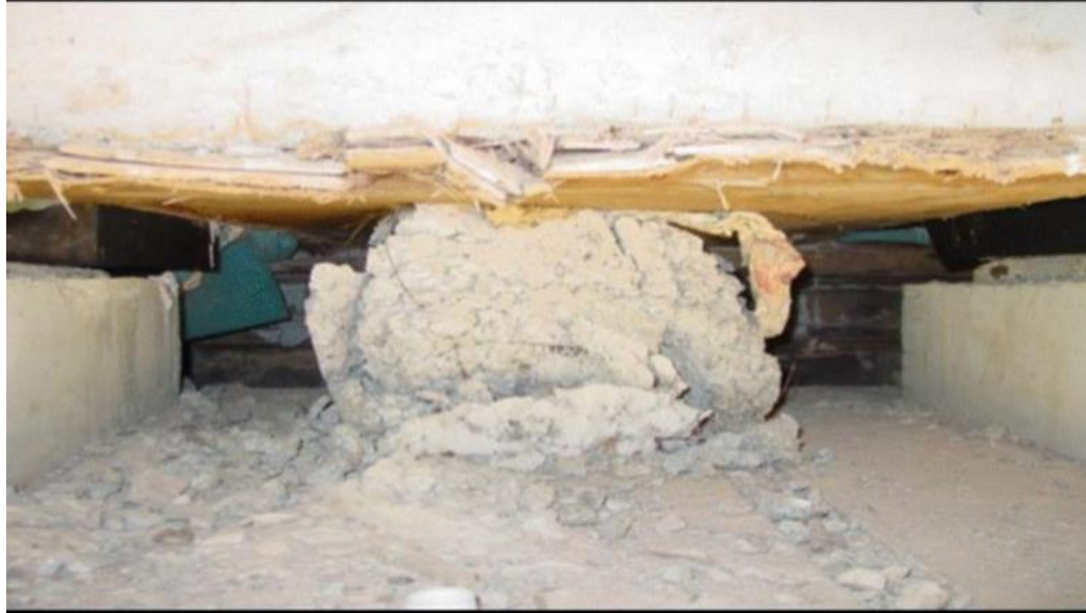
Damaged shear keys
