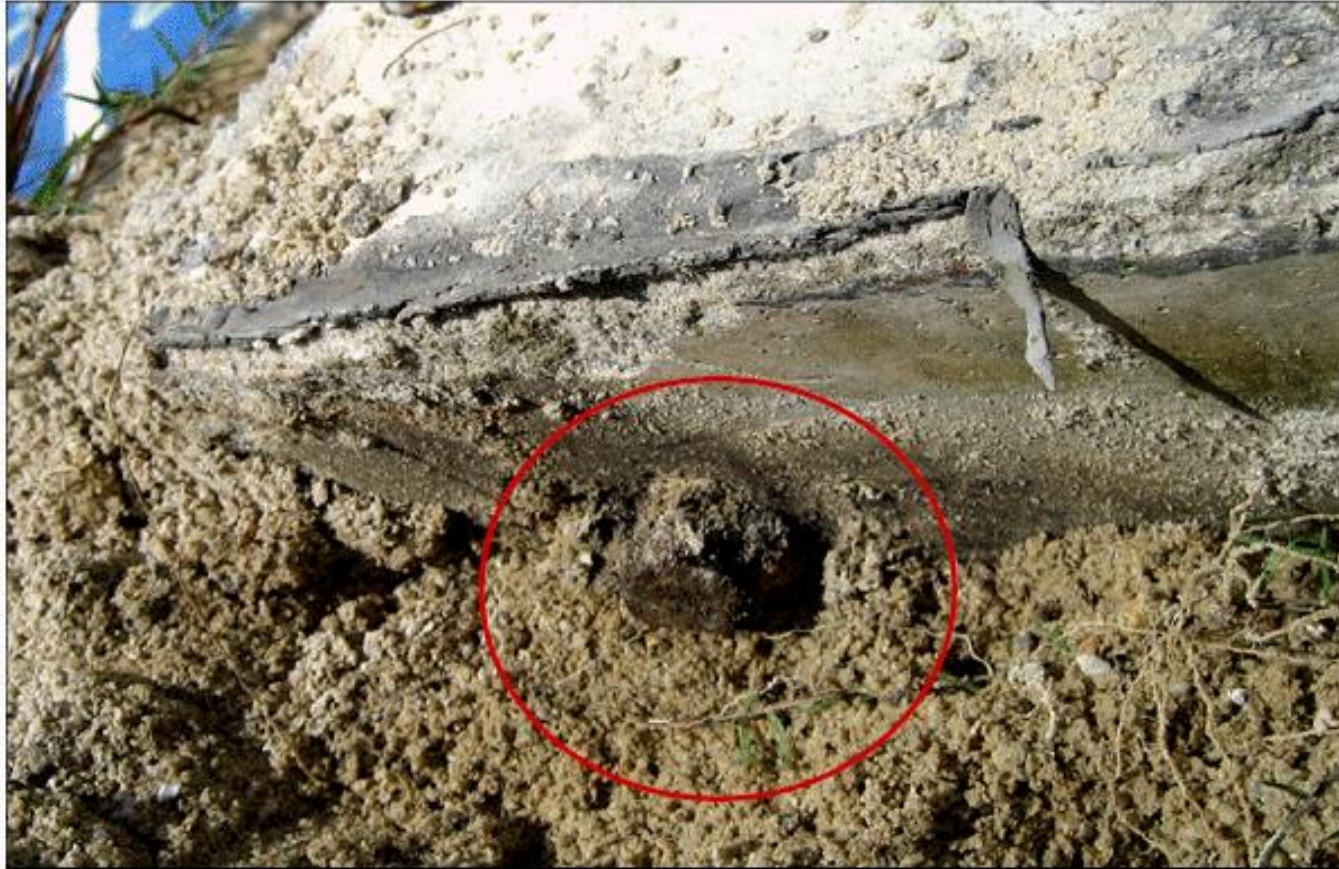
Broken and fractured anchoring bolt of precast parapet
