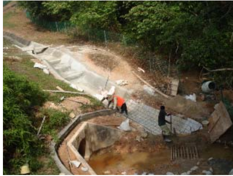
Figure AX2.10: Maintenance Work for Culvert
