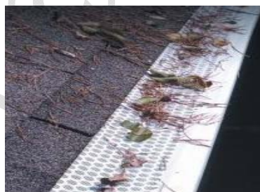
Figure AX2.2: Partially Clogged Gutter Screen
