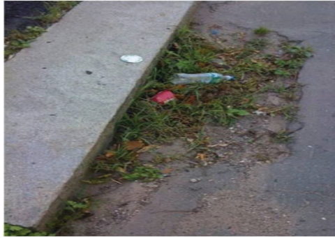
Figure AX2.9: Clogging Inlet
