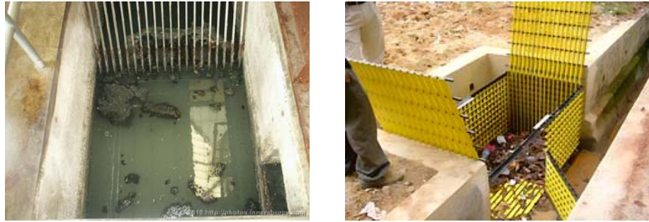
Figure AX2.5: Primary Outlets Clogging
