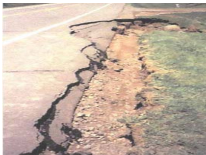
Figure AX2.8: Deterioration of Pavement Edge
