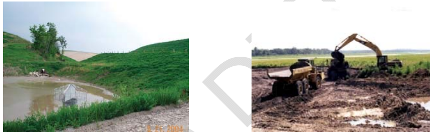
Figure AX2.6: Sediment Removal Work
