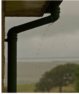
Figure AX2.3: Leaking Downpipe
