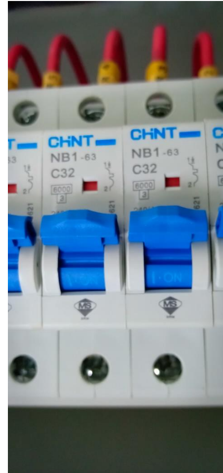
Miniature Circuit Breaker (MCB)
