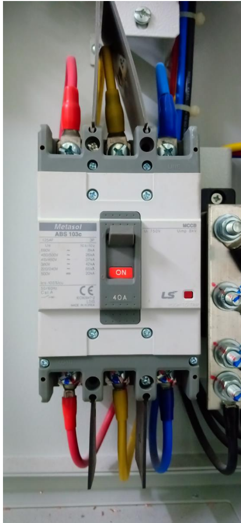
Moulded Case Circuit Breaker (MCCB)
