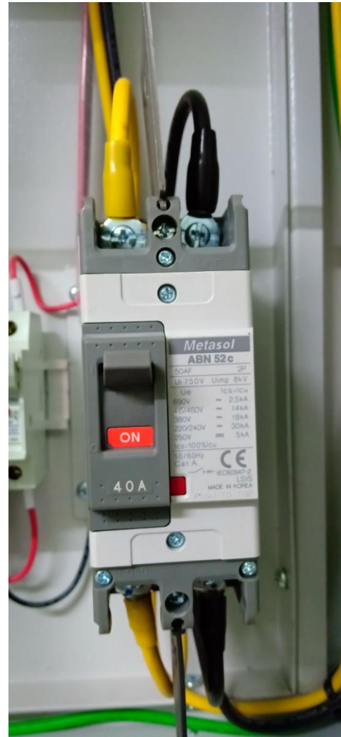
Moulded Case Circuit Breaker (MCCB)
